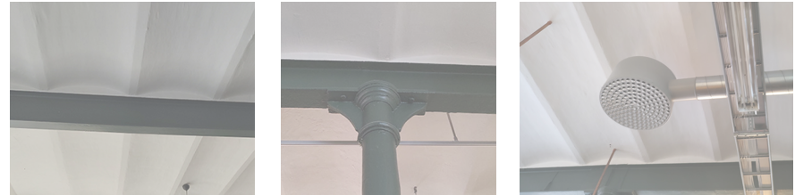
1. Molded vaults, Beams structure and pelars from 1898
