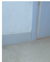
9. Door and wooden details, 1926
