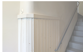
4. Details 1891, original staircase situation
