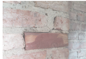
6. Old cracked brick firewall, repaired with wooden bricks
