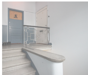
8. Stairs with granite details, 1926
