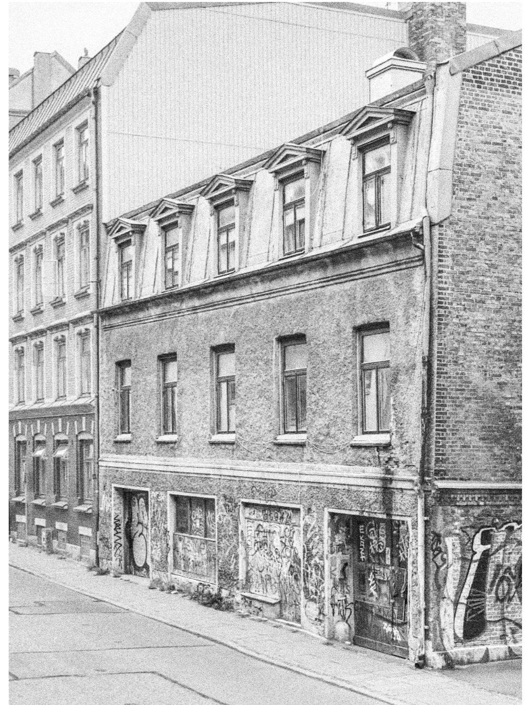
Figure 18. Demolished building, Fjärde Långgatan 9
