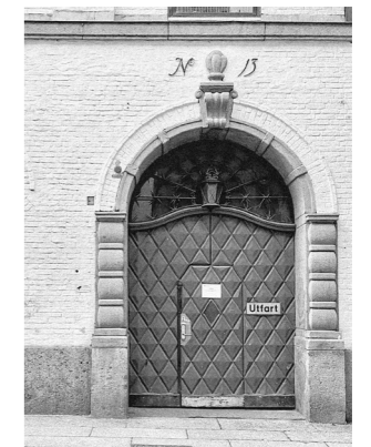
Preserved original entrance, framed by carved natural stone.
