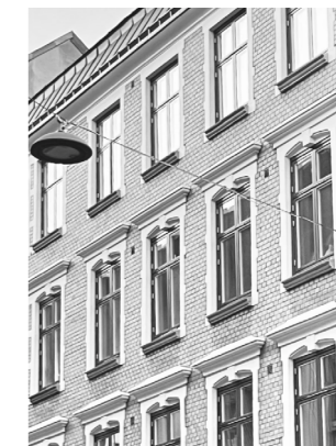
A symmetrical structure of the facade towards the street.
