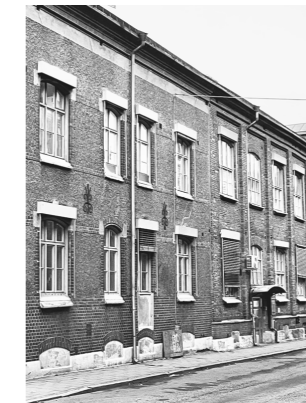
Variation in the exterior illustrate different construction phases.
