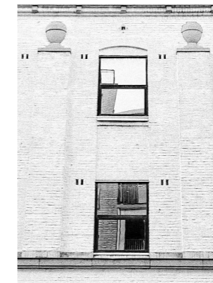
A simple patterned brickwork that follows the arch forms with built-in ventilation hatches.
