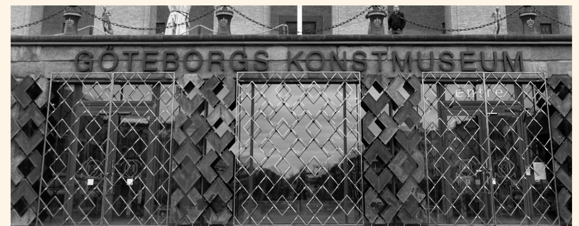
Figure 21: View of the current day main entrance
