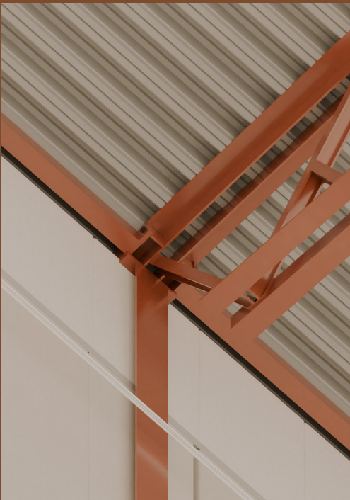
Truss and roof. Ice rink
