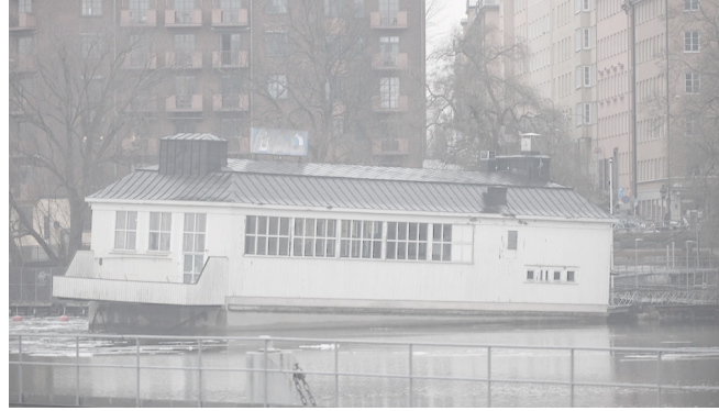
Figure 21. Current situation of Liljeholmsbadhus, shows the corrupted facade and sinking pontoon structure. (Zimmerman, 2023)
