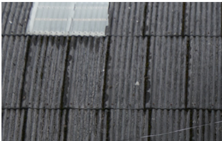
Eternit roof + repair (west)
