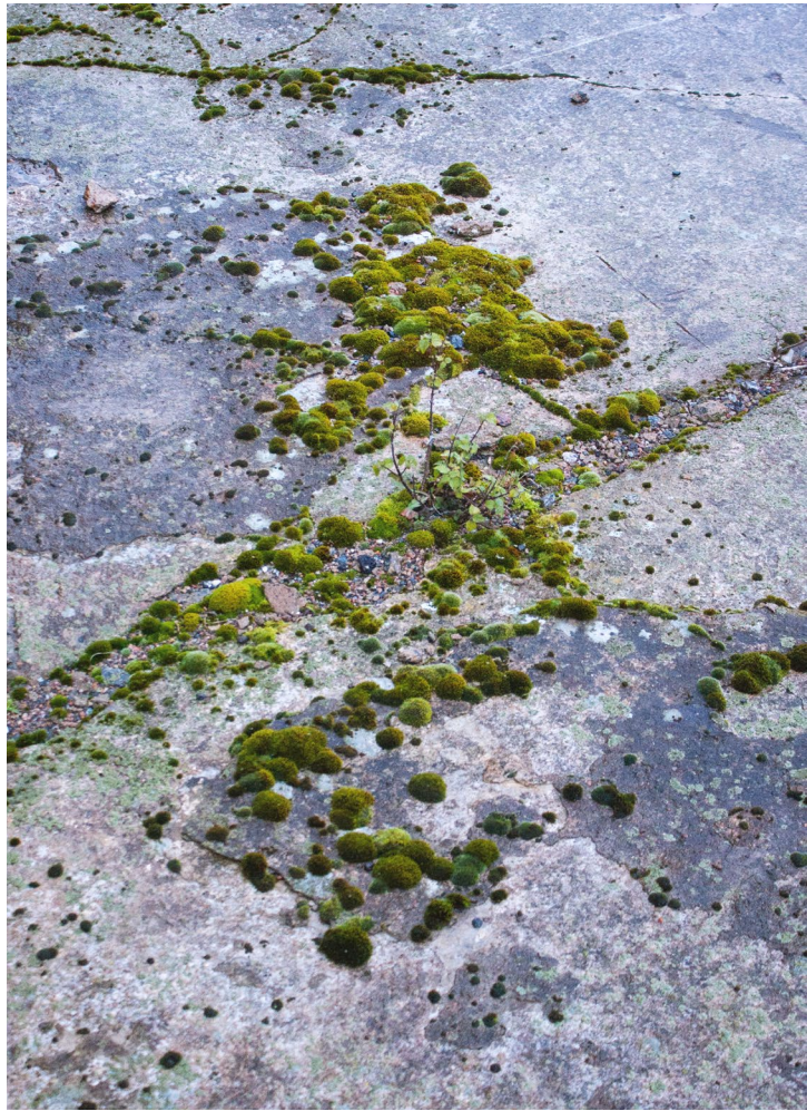
Fig 26. [57.722, 11.989] Moss appears to concentrate and grow along cracks in deteriorating hardscape surfaces.
