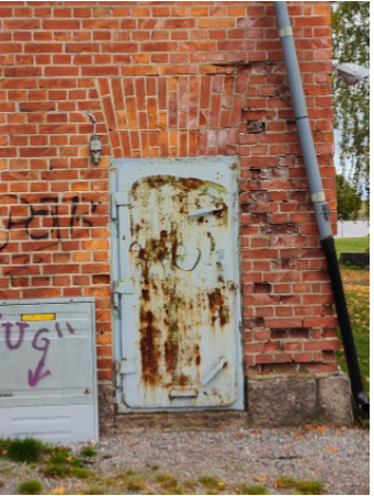
Figure 26. 6. Rusty metal door and damaged bricks
