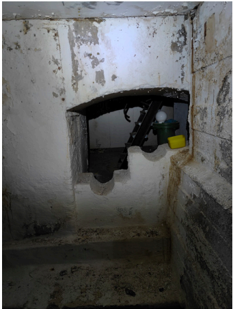
Figure 51. 26. Hole in wall and damaged surface layer
