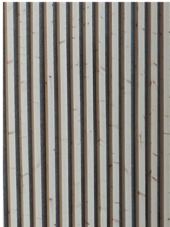
Figure 86. Added pine wood ribs
