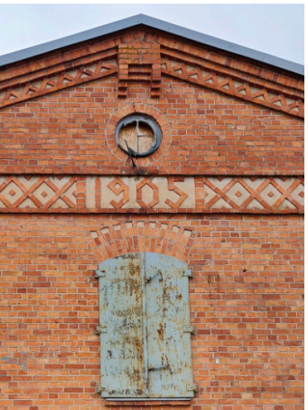
Figure 34. 12. Damaged window frame and rusty shutters
