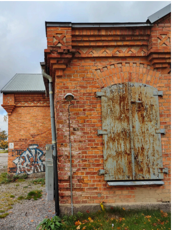
Figure 30. 8. Rusty metal shutter and damaged bricks
