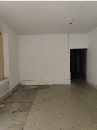
Figure 47. 23. Metal hatches in concrete floor and cable remains in ceiling
