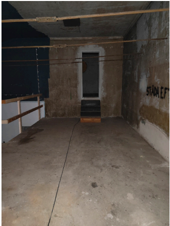
Figure 37. 14. Loose tie rods and height differences
