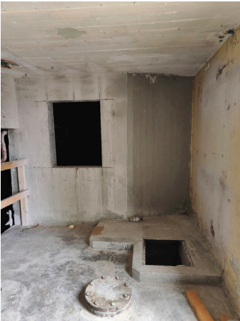
Figure 43. 19. Cisterns and an opening in the floor, surface layers in poor conditions
