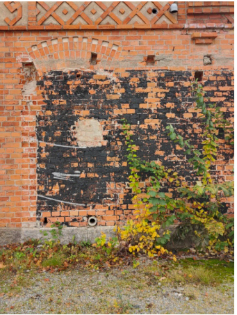
Figure 24. 4. Dark coating and arches suggesting earlier window placements
