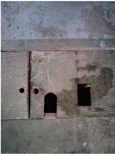
Figure 16. Metal hatches in floor
