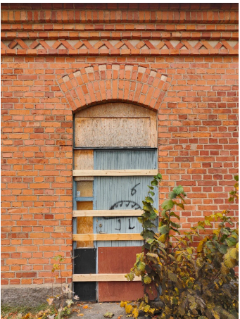
Figure 33. 11. Wooden door with broken glass partitions
