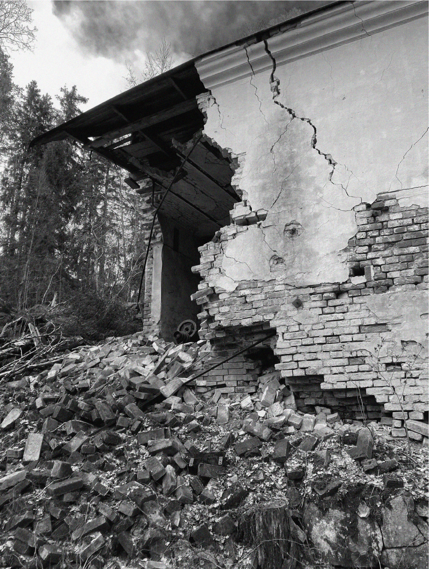
Figure 22: Hole north facade
