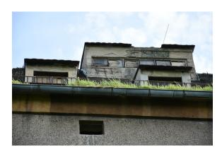
Figure 12 Grass growing on the roof of the silo May 2022
