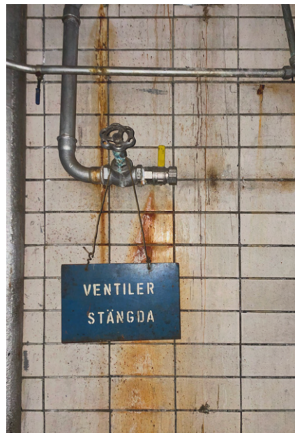
A very dirty part of the boiler room wall, subject to staining and burns, before the application of latex.
