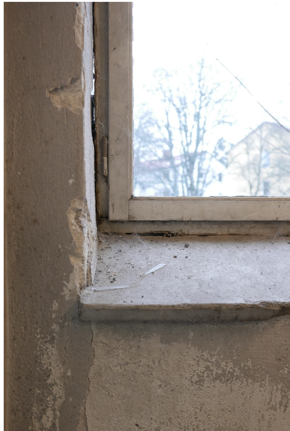
Deterioration of wall and window in the pump room
