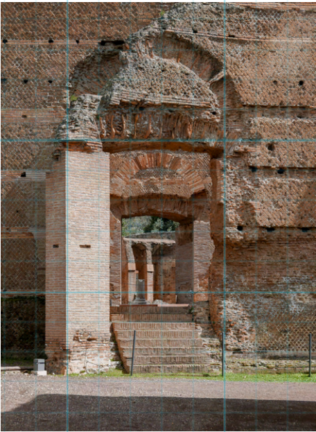
f11: Reconstructed archway at Villa Adriana in Tivoli. The reconstruction follows the principle of differentiation. Authors’ photograph.
