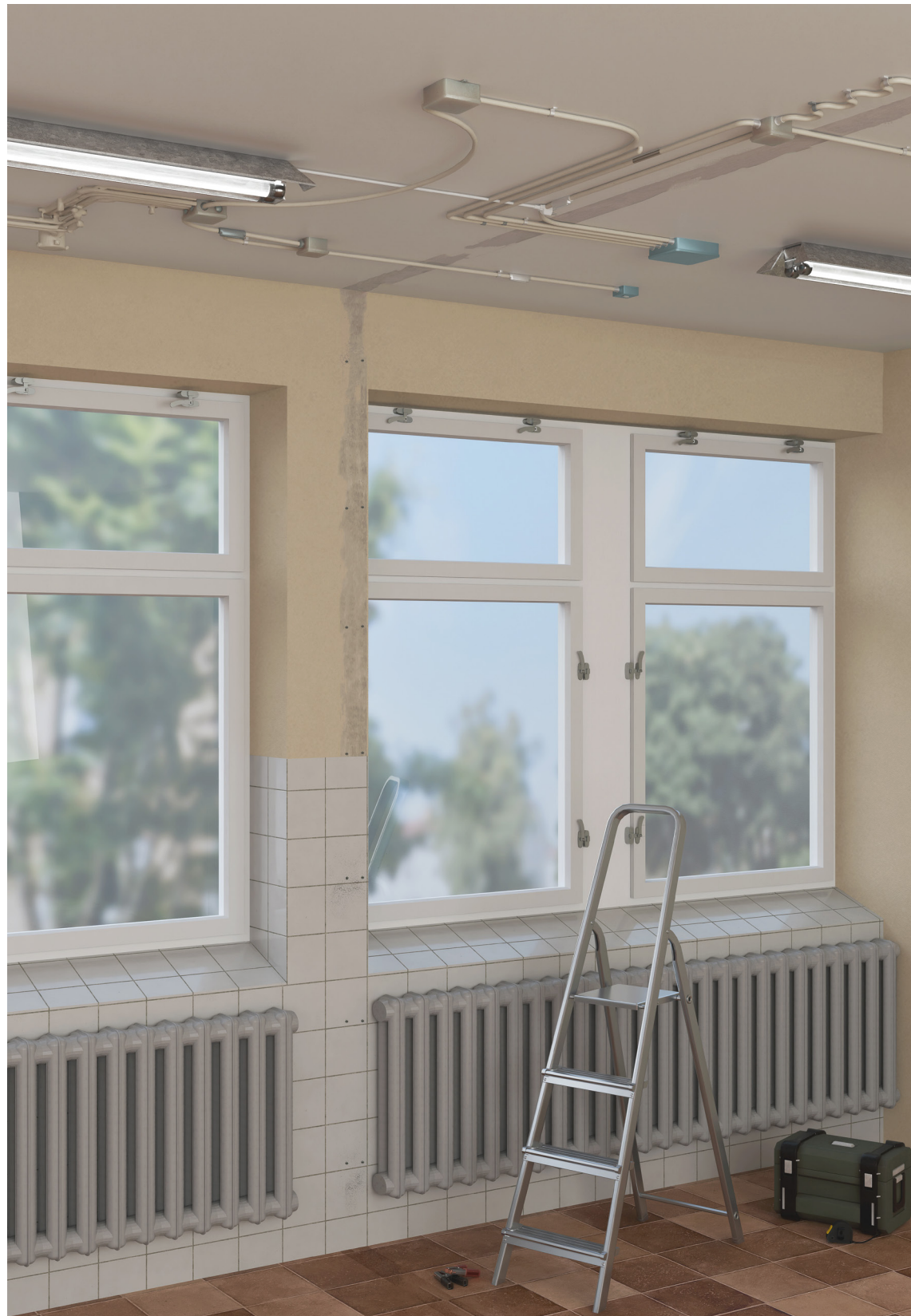
fig. H Assembly of electrical artifacts in the laundry room in progress. The previous wall dividing the room has been removed, leaving a visible trace in the wall and ceiling.
