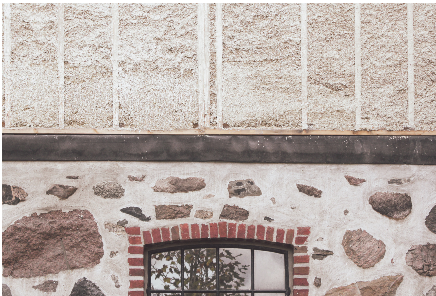
sprayed hempcrete on a timber structure
