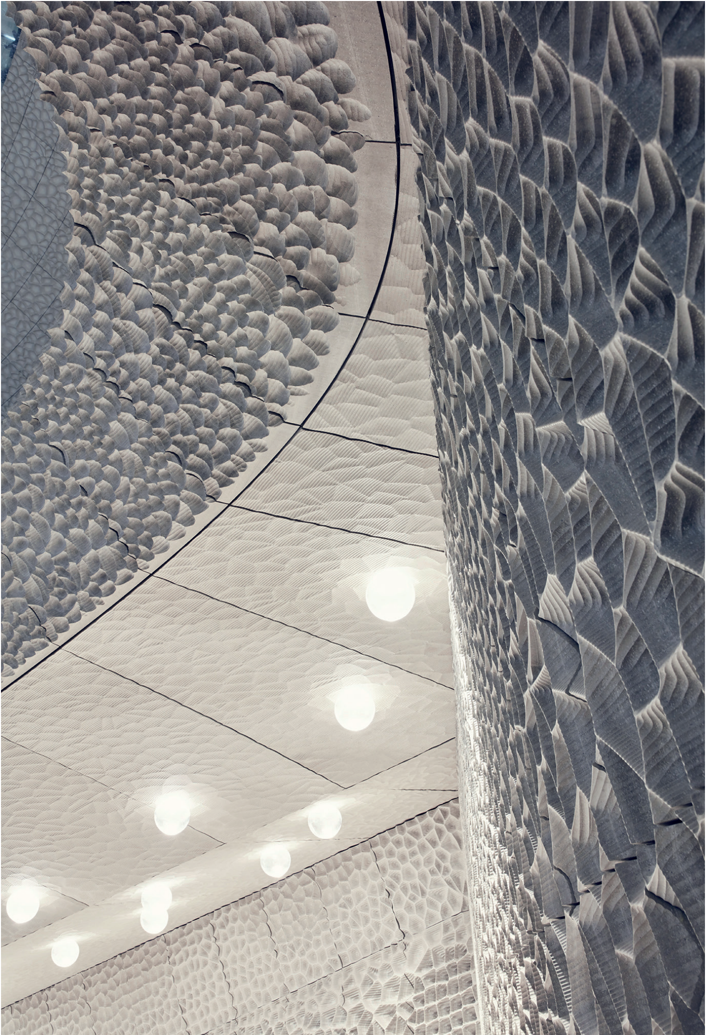
Figure 4 - Photograph of custom developed gypsum panels (Schulz, 2023). Reproduced with permission.
