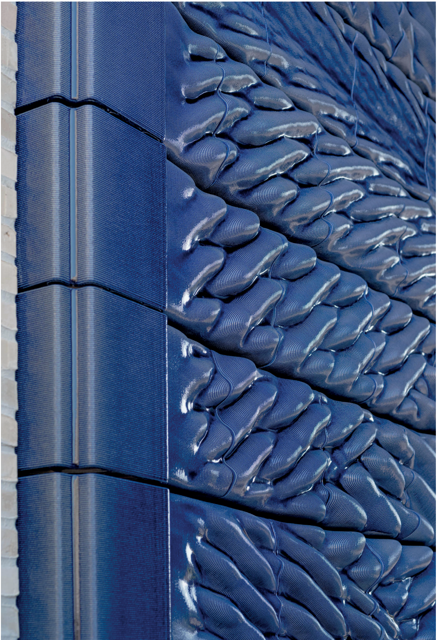
Figure 3 - 3D-Printed clay fused with artisanal glazing (De-Vecchi, 2023). Reproduced with permission.
