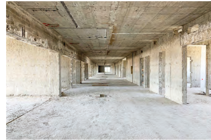
F26: Stripping phase photograph of conversion of the Felix Platter Hospital in Basel (ARGE Müller Sigrist Architekten, 2022). This photo distinctly demonstrates the raw concrete beneath the dismantled surfaces.
