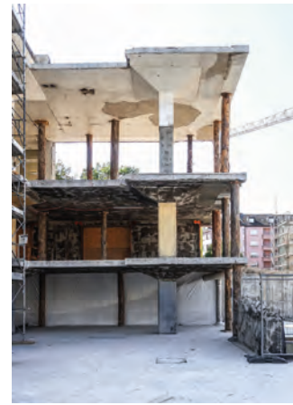
F22-24: Left: Concrete mushroom pillars highlighted in the middle of the room. Above: The stripping phase reveals the stacking of the mushroom pillars evidently in different heights. Above: The cross section is showing the original structure in black and additions in red.
