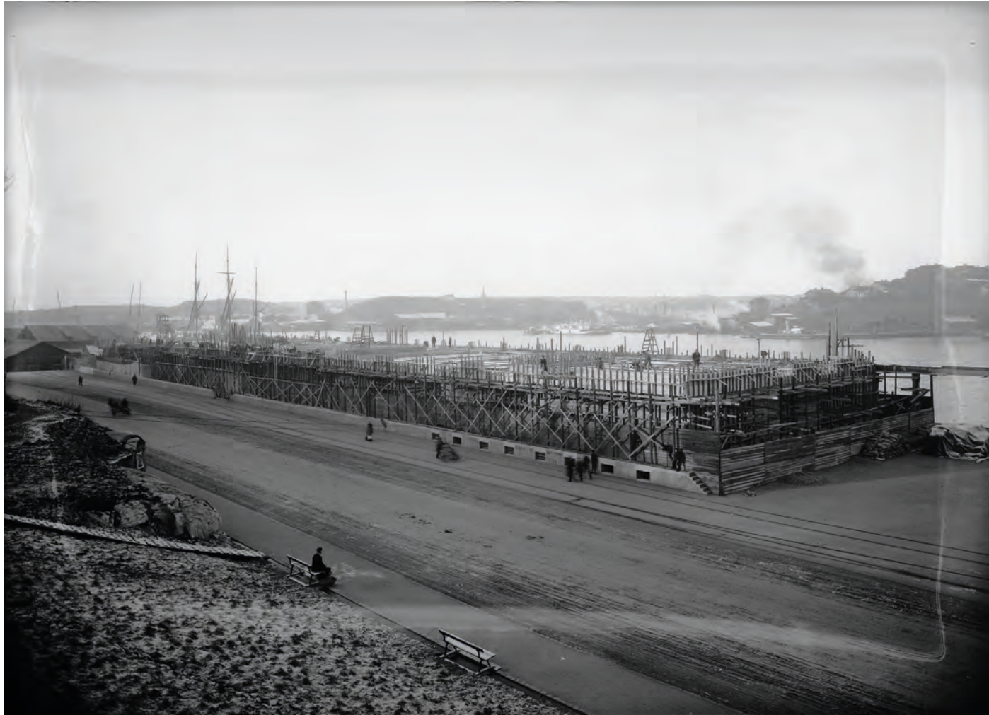
F33: Construction of Amerikaskjulet, using timber to cast the concrete. In the background, smoke can be seen from the industries of the harbour in Sannegården. It is evident that the maritime industry contributed to a completely different skyline than today.
