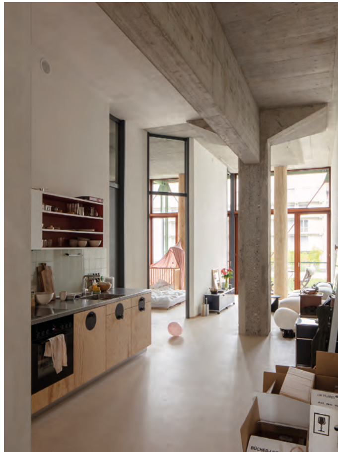
F22-24: Left: Concrete mushroom pillars highlighted in the middle of the room. Above: The stripping phase reveals the stacking of the mushroom pillars evidently in different heights. Above: The cross section is showing the original structure in black and additions in red.
