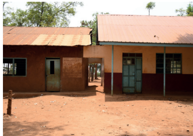
28 Path between 3rd, 4th and 5th grade buildings
