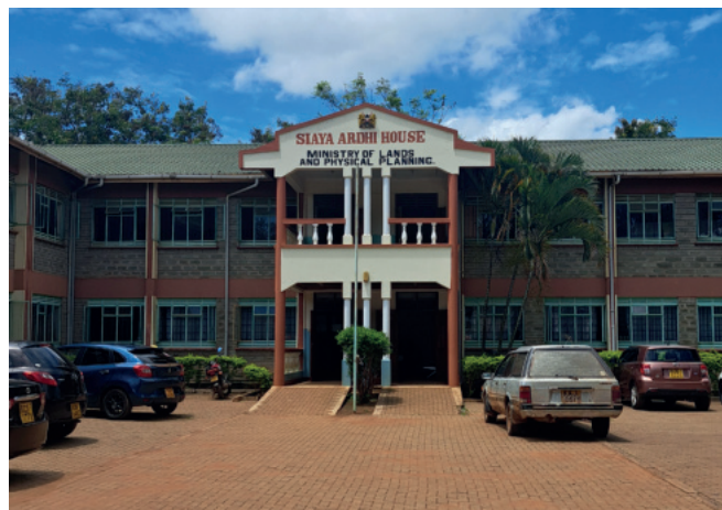
Building Ministry of lands and physical planning
