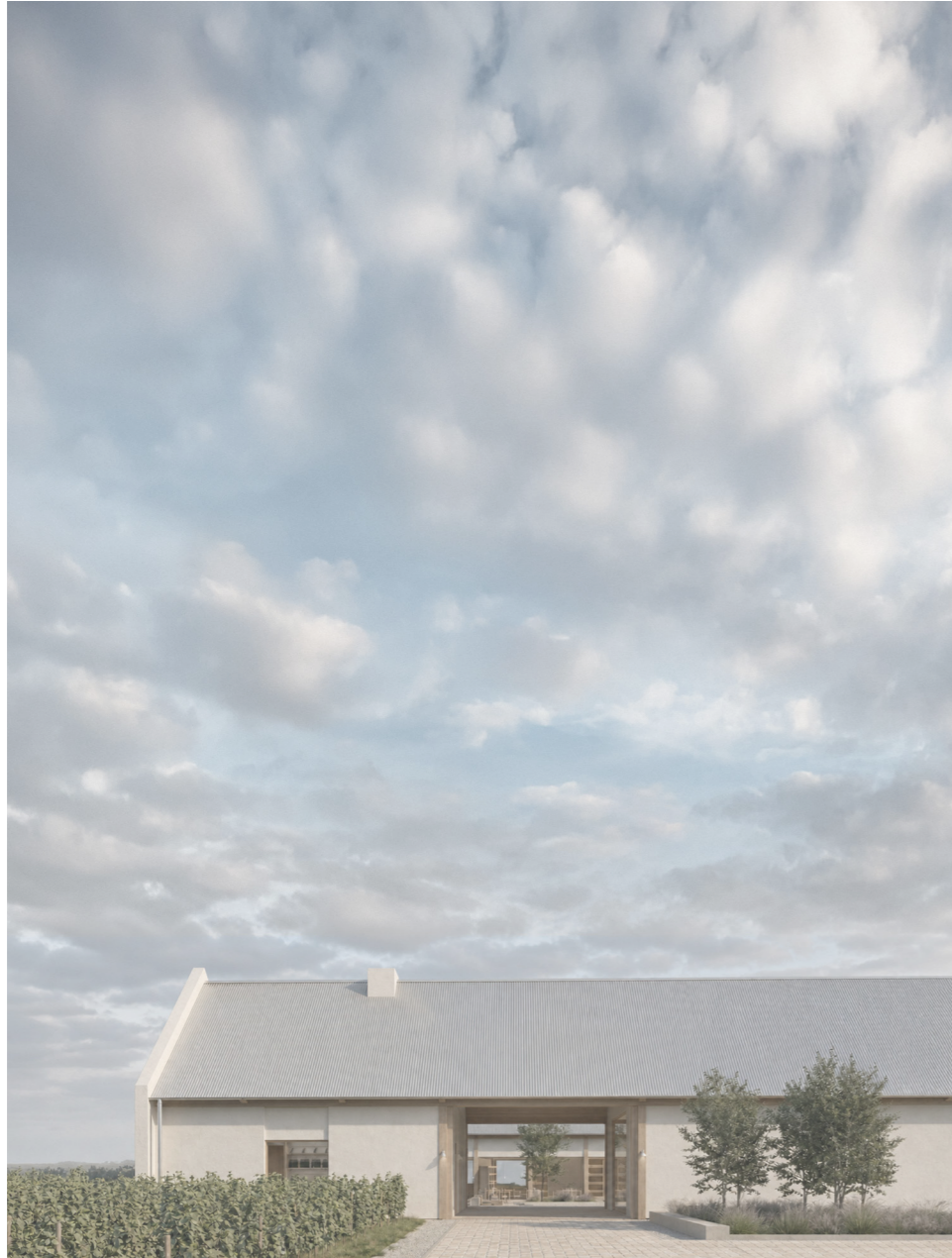
Approaching the building.
