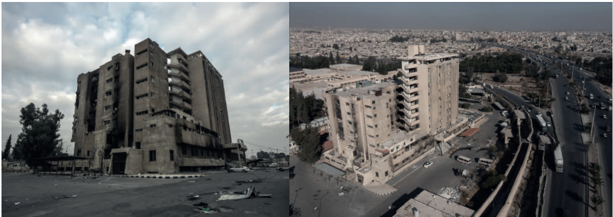
Figure 75. Exterior views of the Palestine Branch (Branch 235) building in Damascus, various views. Source: Adapted from Al Jazeera Website.
