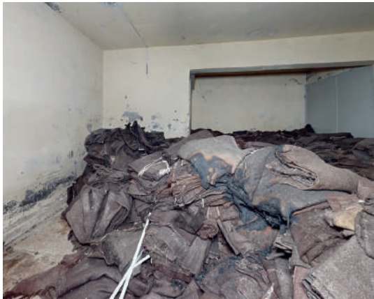
Figure 34. Traces of fire in “Cell 1 – A Left”, third floor. Source: Adapted from Syrian Prisons Museum.
