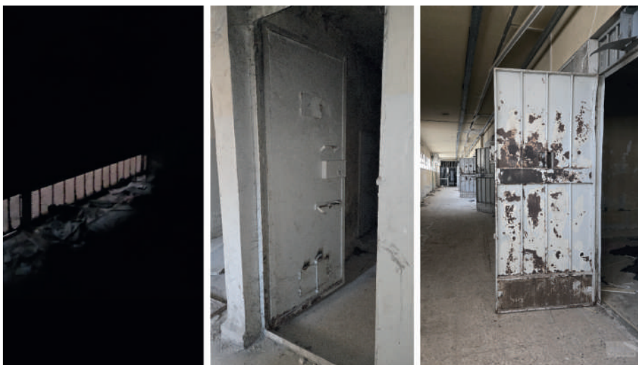
Figure 38 . Field visit photographs illustrating how the design of the cell doors severely limited access to natural light, contributing to the darkness experienced inside the detention spaces. Source: Author.
