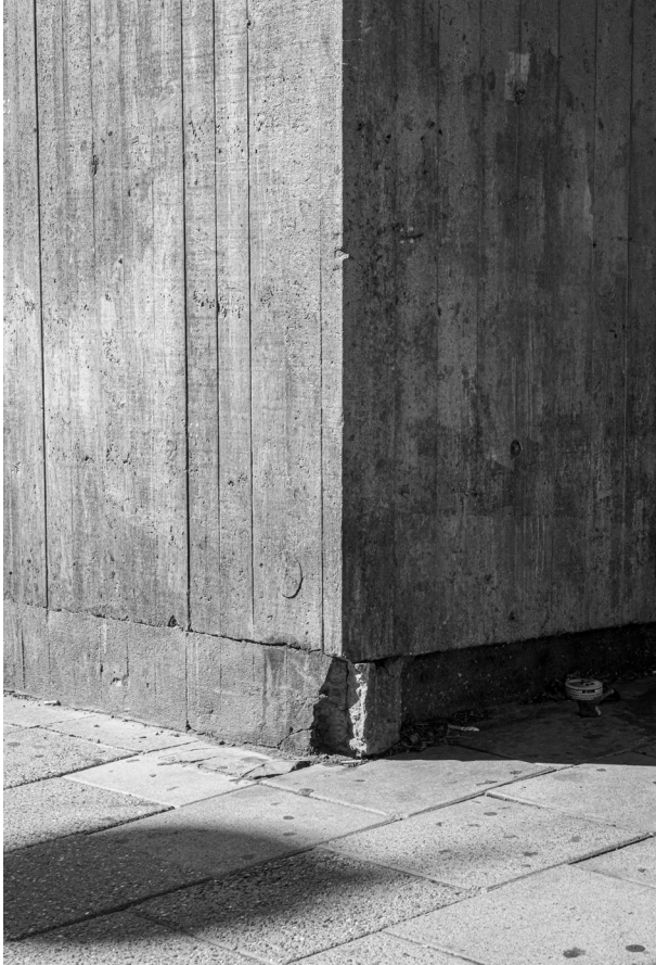
Fig. 35 Trace of ageing, concrete crack. © Inès Romy
