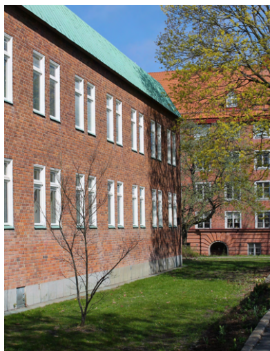
h. Southeast facade
