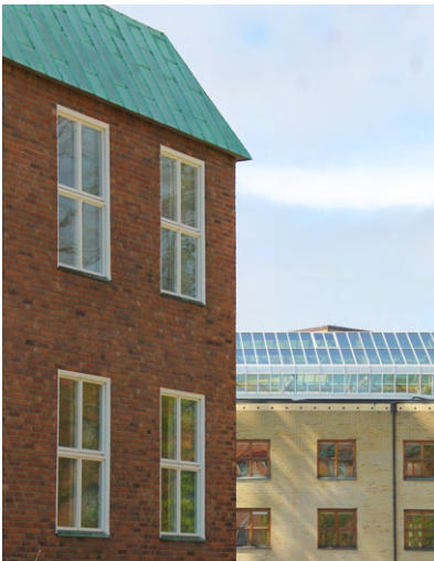
d. Meeting facade - roof (SE)
