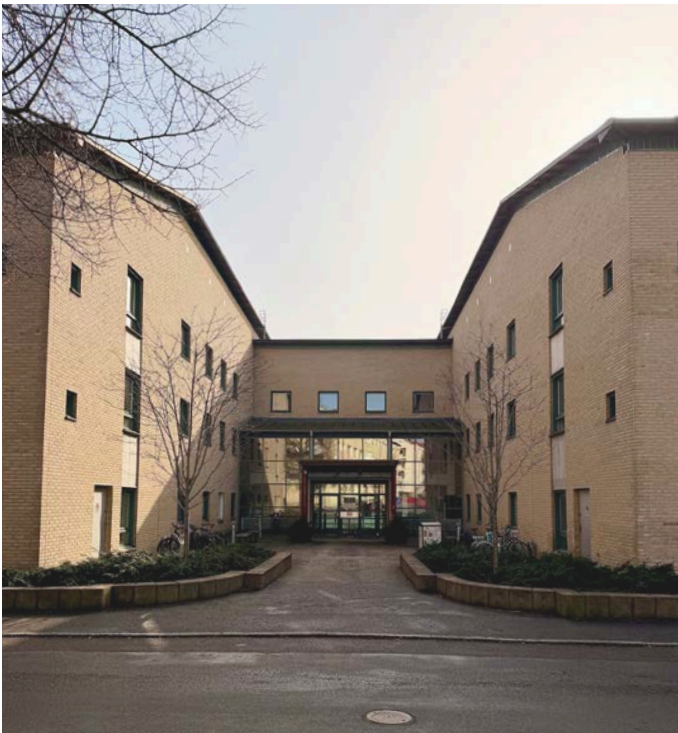
Figure 17: Eklandagatan 86, entrance from the north side, main entrance (2nd floor)
