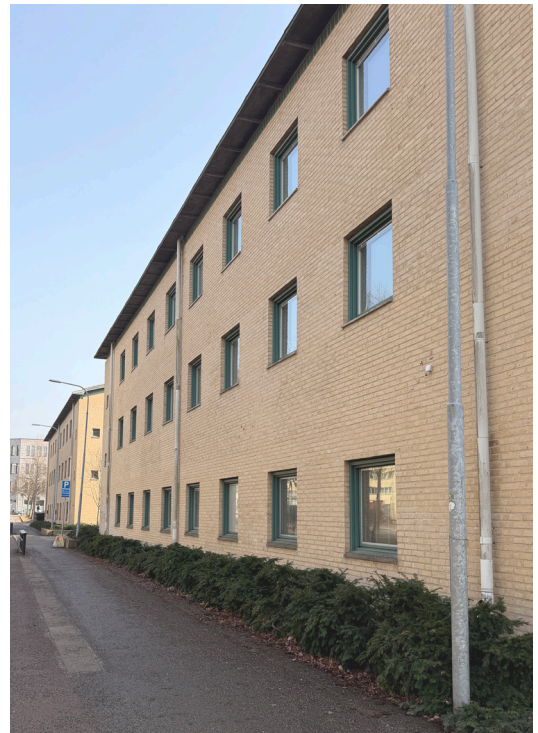
Figure 18: Eklandagatan 86, connection between street and entrance level (2nd floor)
