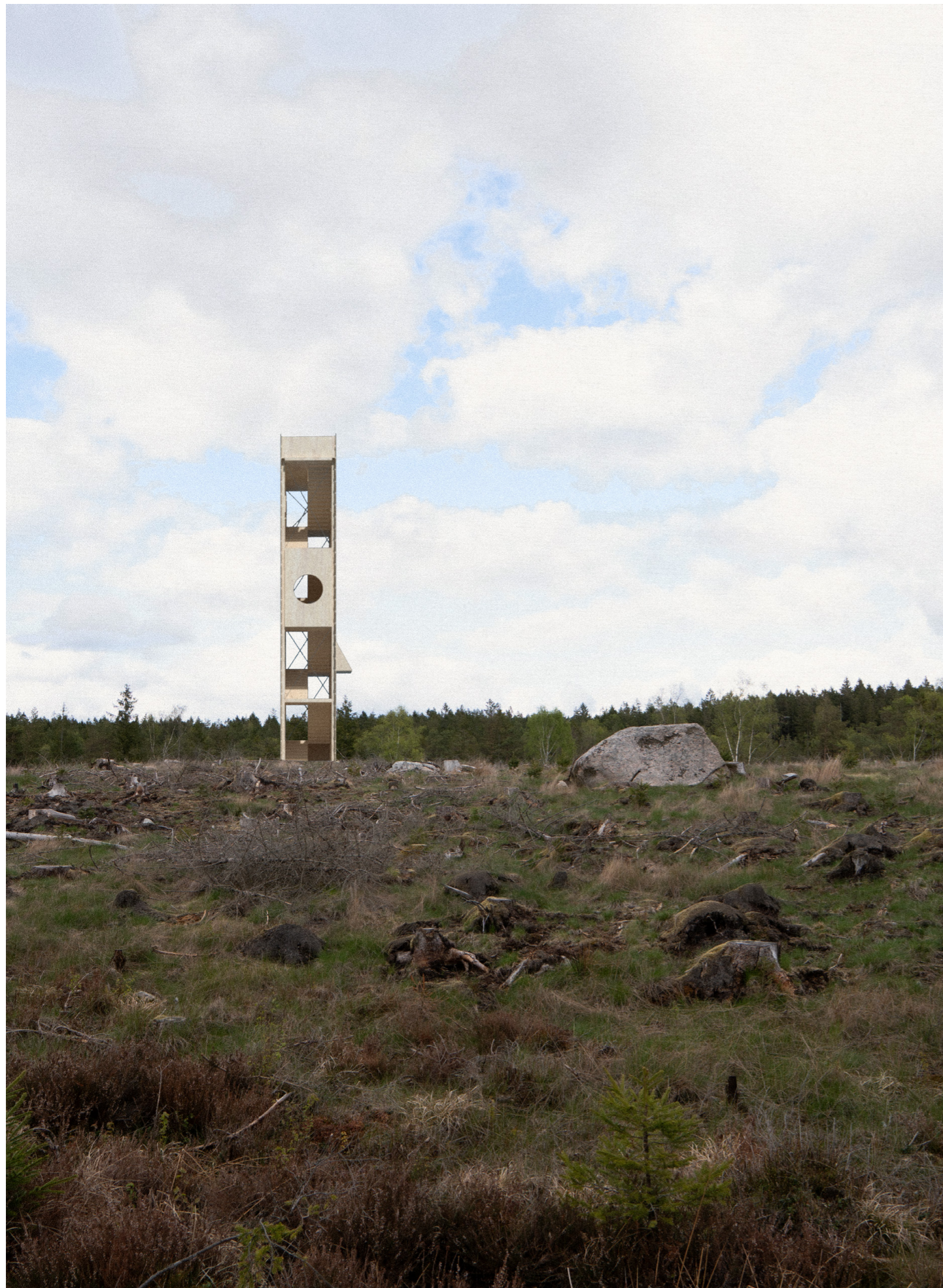
Exterior perspective of the Tower. The Tower rises above the perimeter of the clear-cut.
