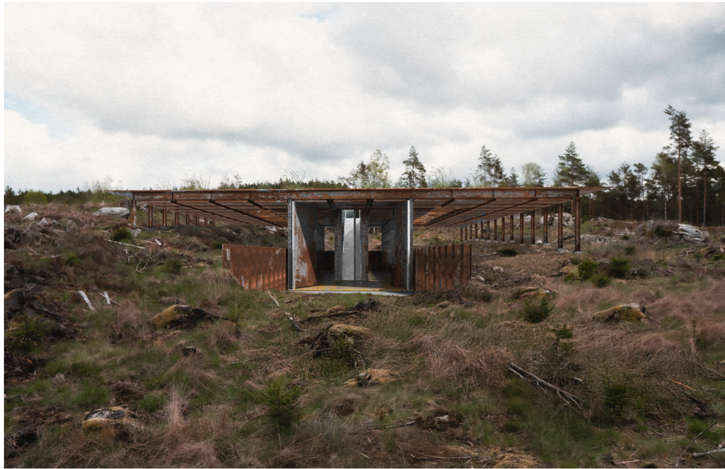
Exterior perspective of The Exhibition. The staircase of the exhibition hall guides the visitor up onto its roof.
