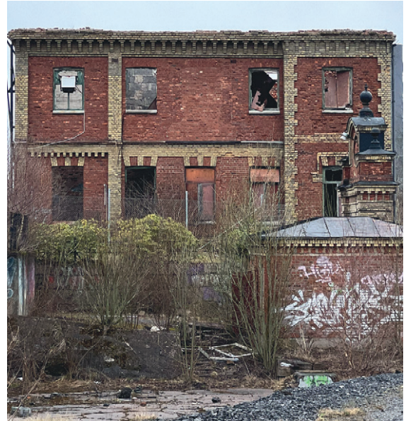
Figure 24. Photograph. South facade.
