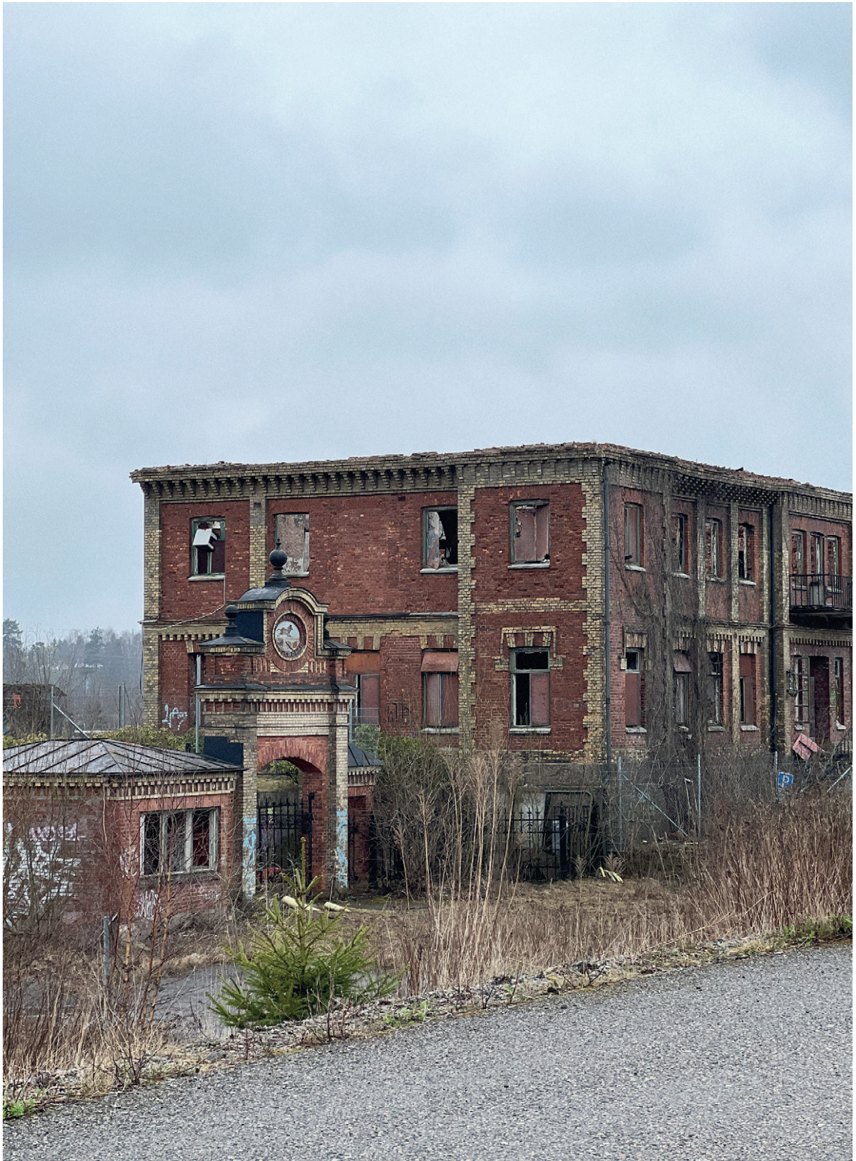
Figure 20. Photograph of the old office.
