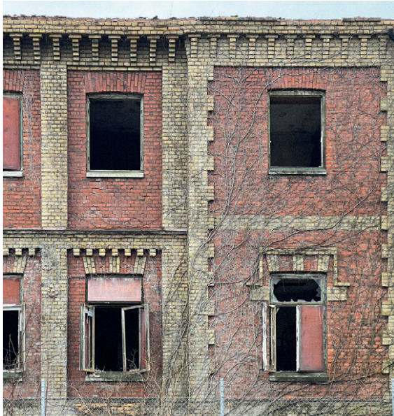
Figure 27. Photograph. Part of east facade.
