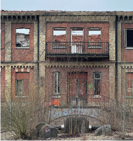
Figure 21. Photograph. Part of east facade.
