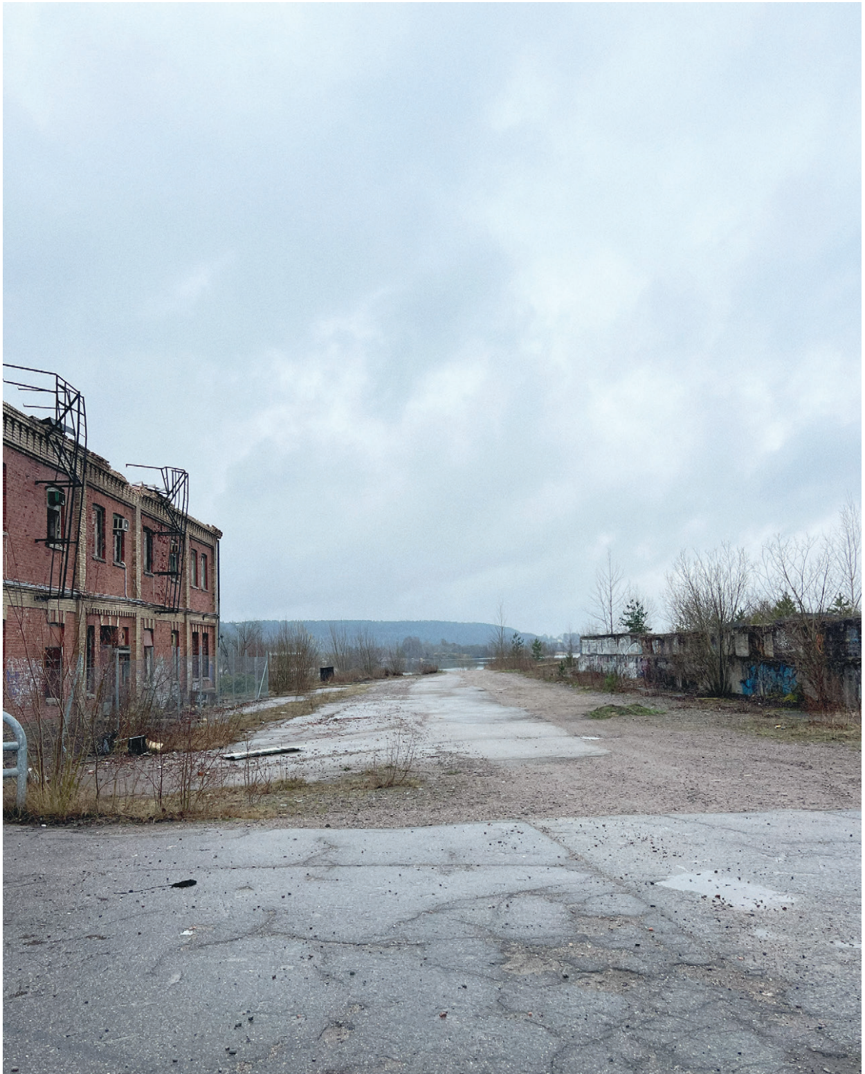
Figure 34. Photograph of the site and west facade of old office.
