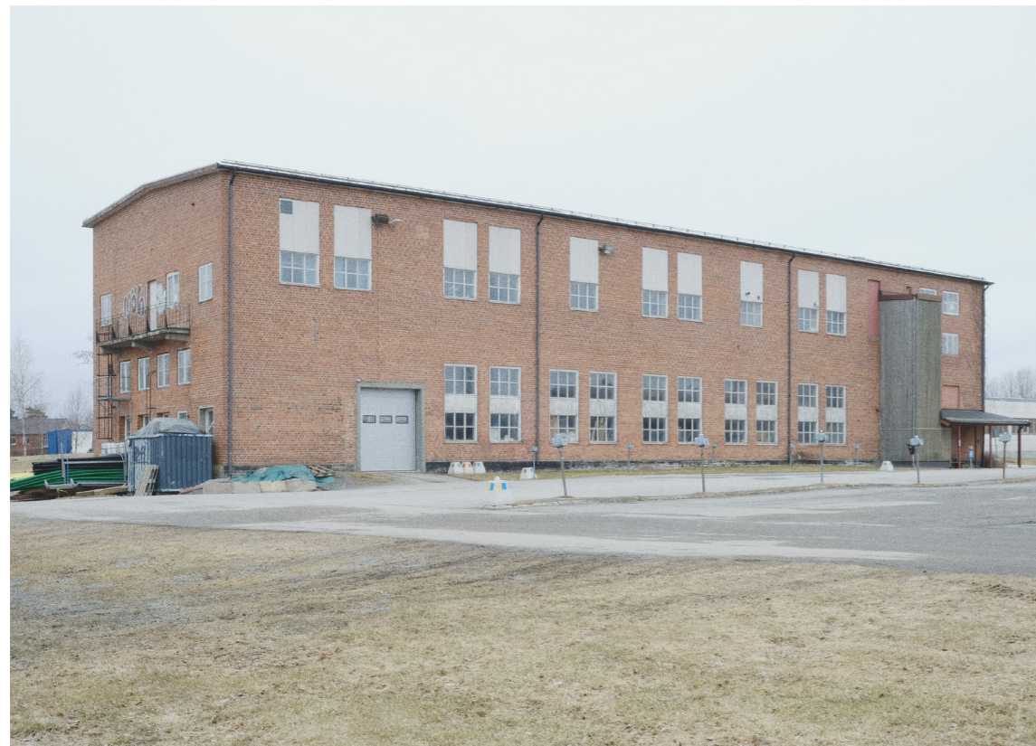
Photographs, existing condition of exterior
