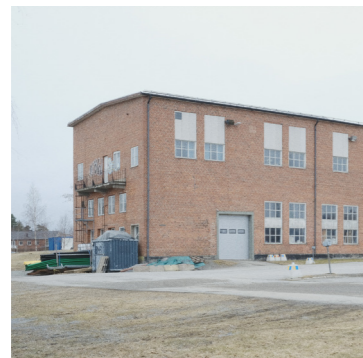
Photograph, current state
