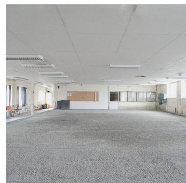
Photograph, current state
