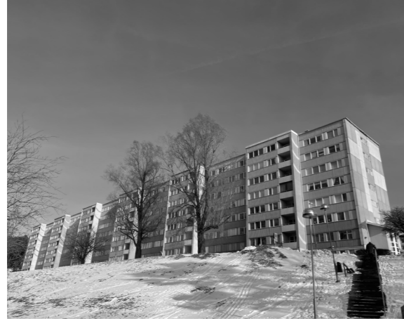
Figure 2: Housing Block at Siriusgatan
