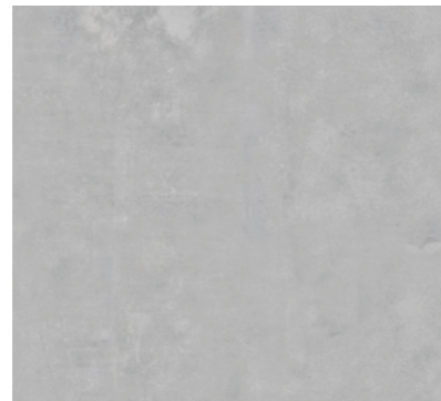
Concrete ground in atrium
