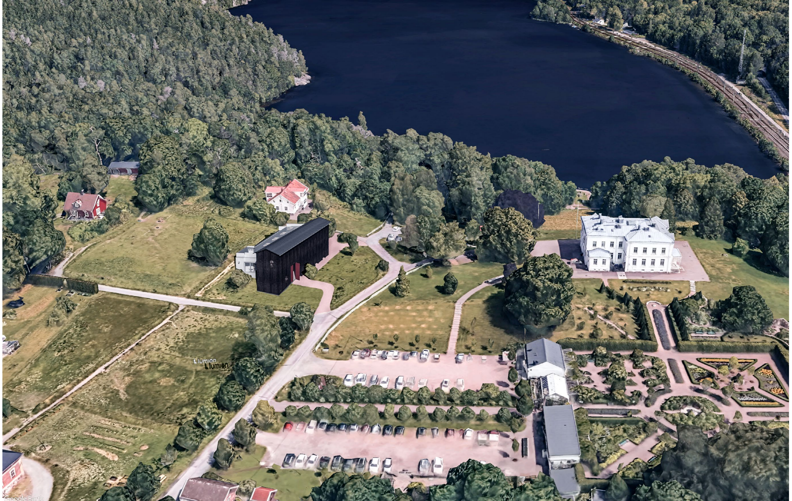
Fig 21. Overview of site and project.
