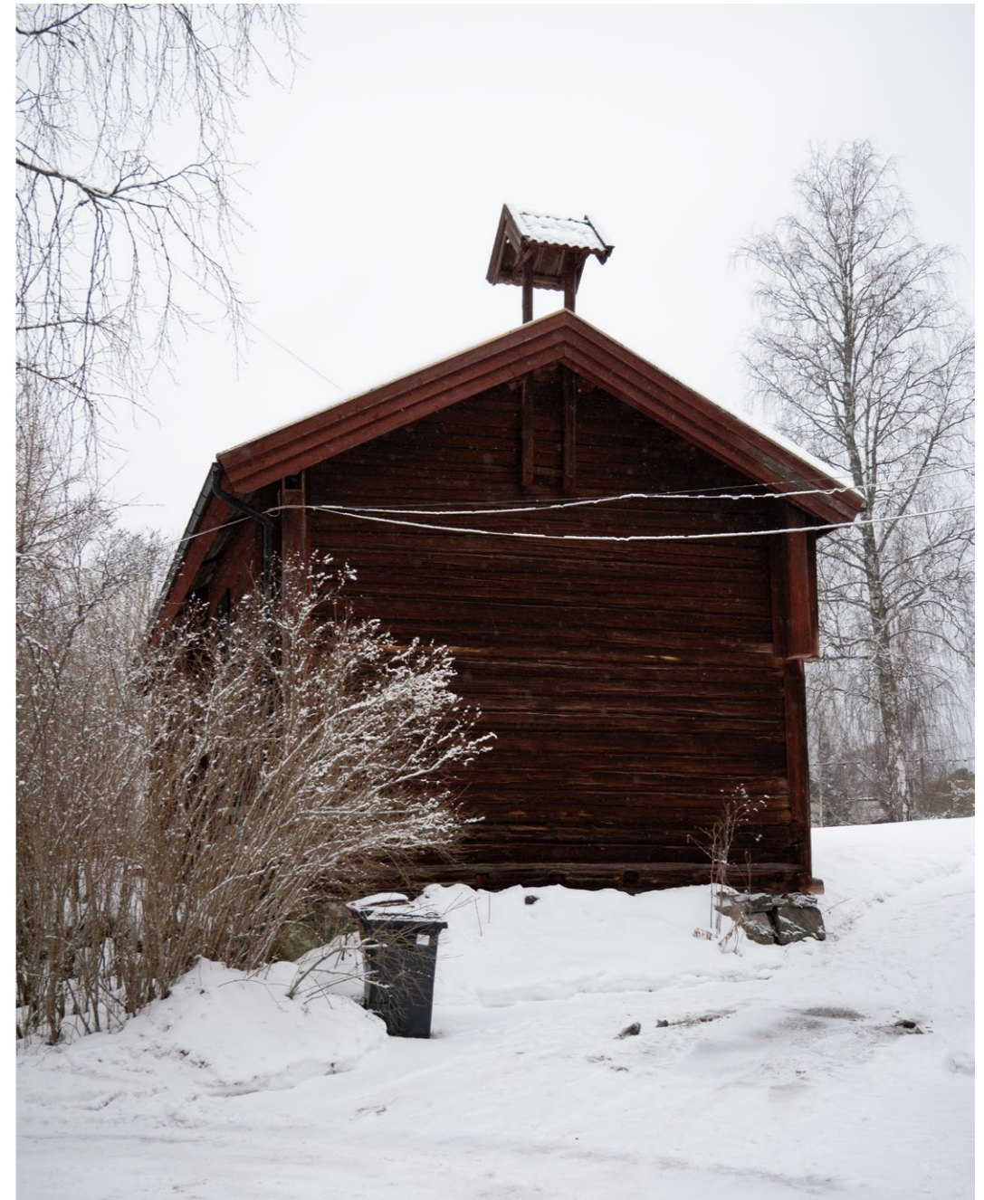
Fig 20. Storage building in Stora Hyttnäs.
