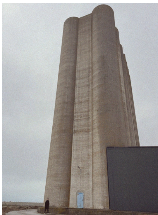
Figure 31. Photograph of east facade.
