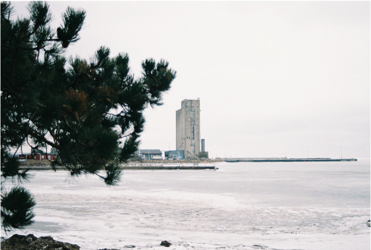
Figure 24. Exterior view, south beach point.
