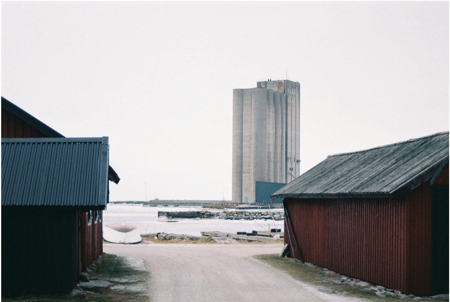
Figure 23. Exterior view, north fishing point.
