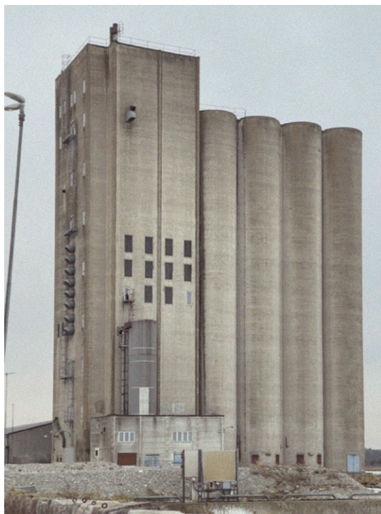
Figure 28. Photograph of south facade.
