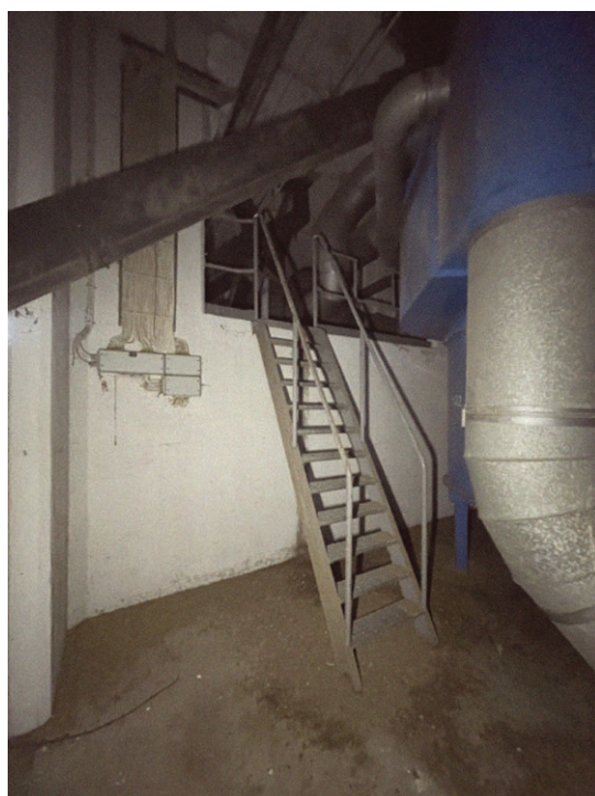
Figure 37. Interior photograph, mezzanine.
