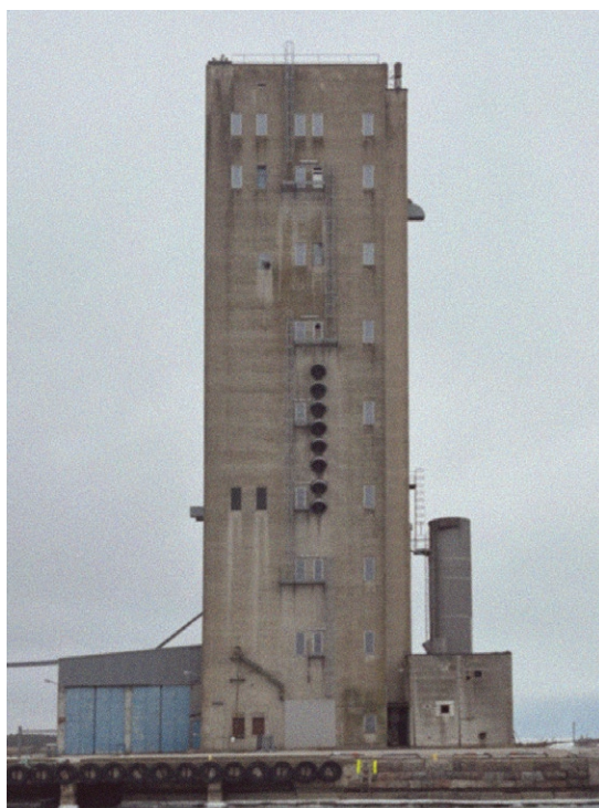
Figure 30. Photographs of west facade.
