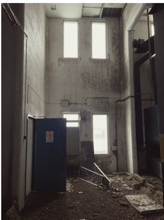
Figure 36. Interior photograph, corridor windows.
