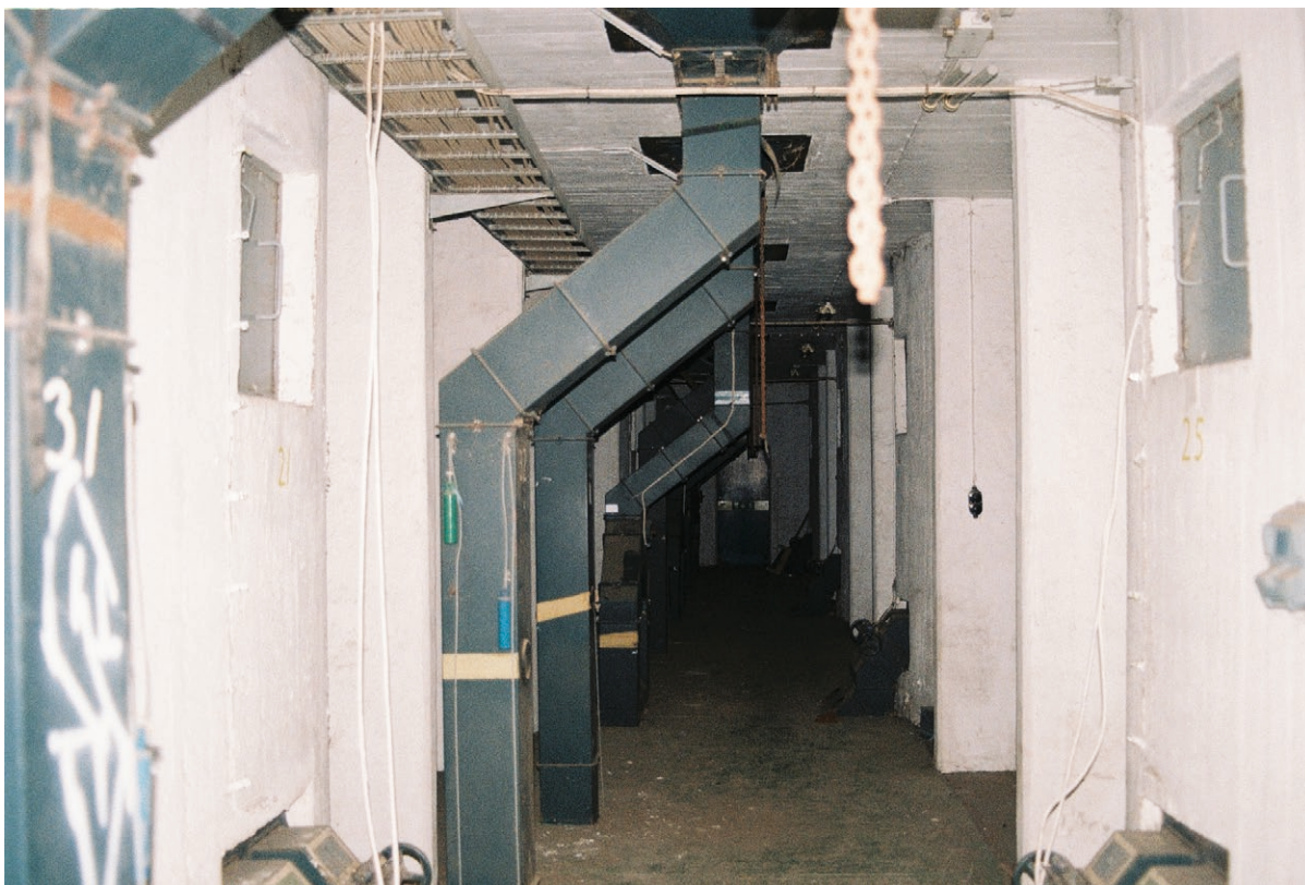
Figure 39. Interior photograph, center corridor.
