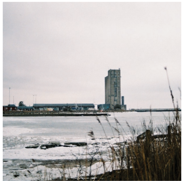
Figure 18. Exterior view, south beach point.
