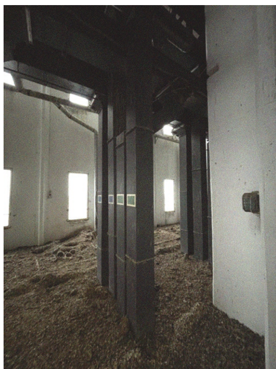
Figure 41. Interior photograph, existing light intake.
