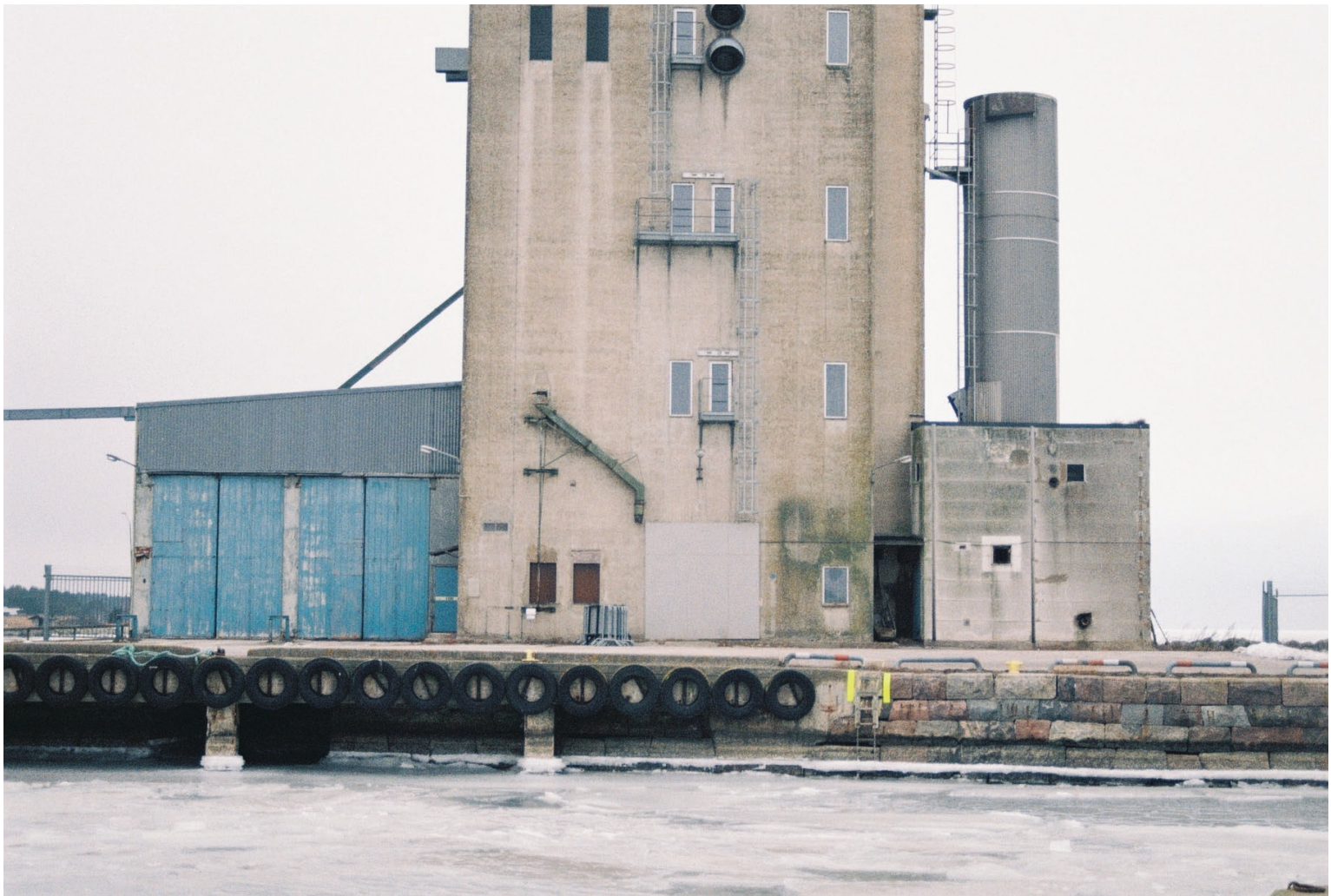
Figure 25. View on west facade.
