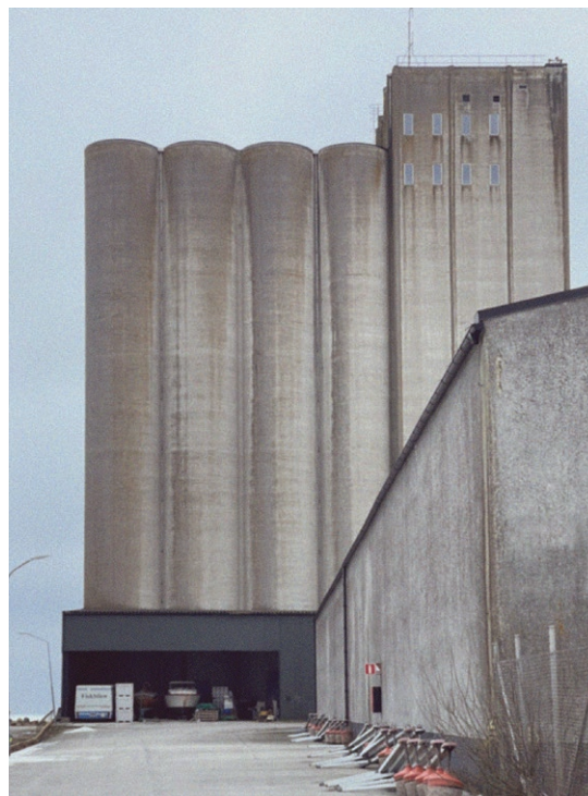
Figure 29. Photograph of north facade.
