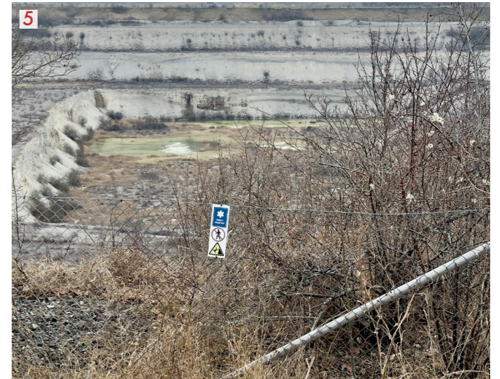
Fig 12 : protected quarry edge and restricted access
