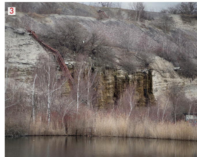
Fig 10 : Water pump pipe and vegetation along cliff edges
