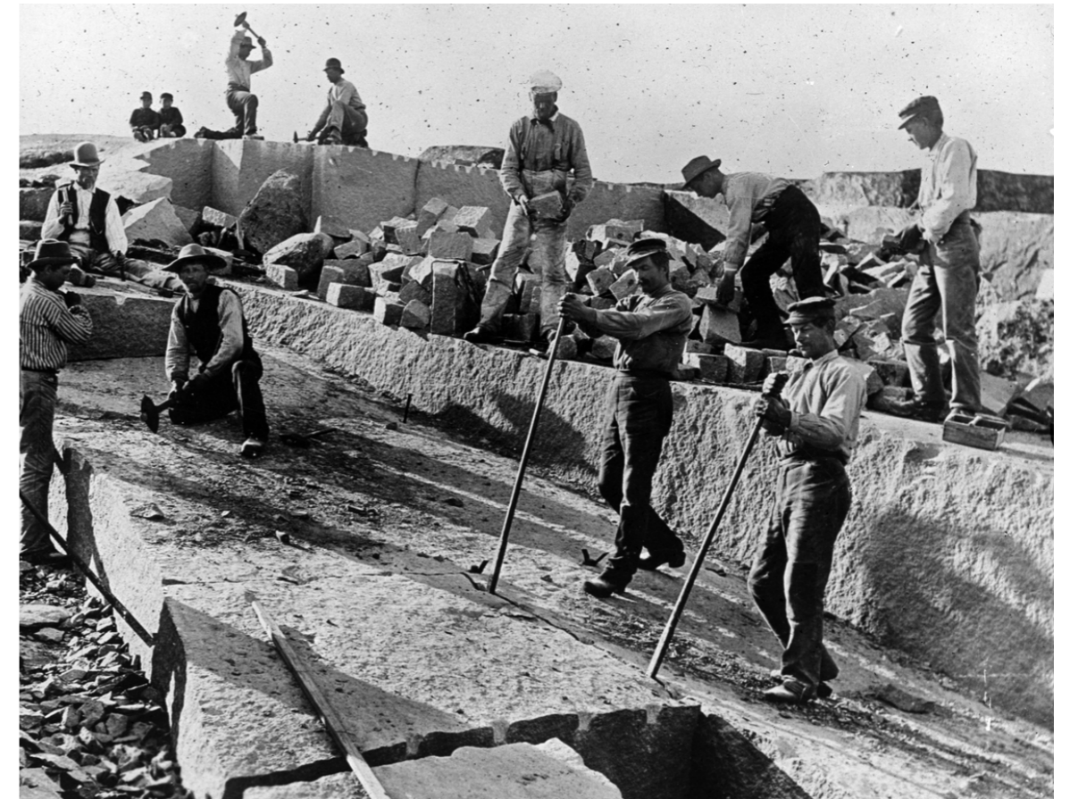
Fig. 6 Figure X. Photograph of stonecutters working on Bohus-Malmön, Sweden (UMFA54695:0036). Public domain.
