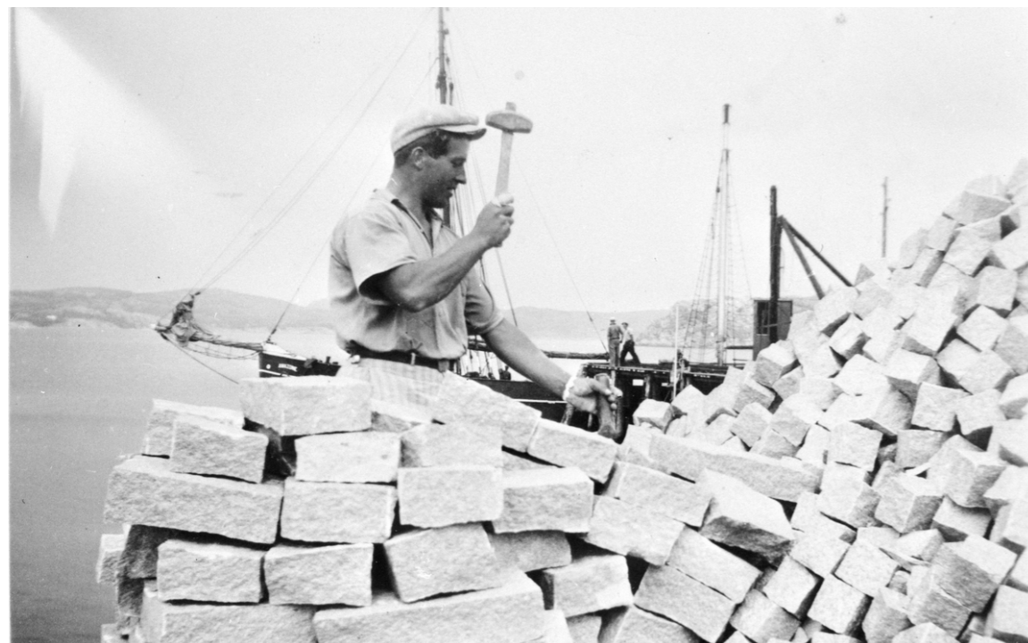
Fig. 5 Photograph from Bohusläns museum (UMFA53014:0021), depicting a stonemason cutting paving stone. Public domain.
