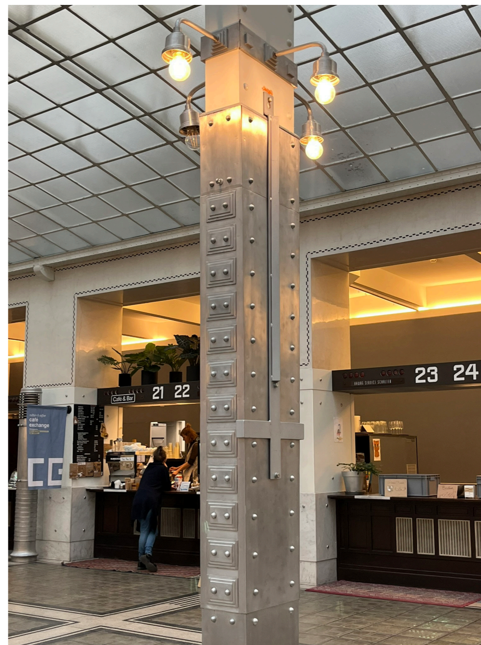
column detail in grande cashier hall (café exchange in the background)
