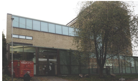
Gothenburg Museum of Art - East Etagera - 4 Falkhallen - 5
