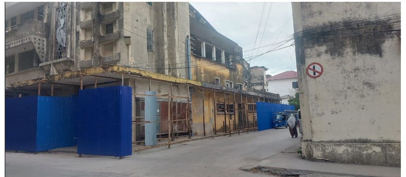
Fig.15 Majestic Cinema scaffolding
