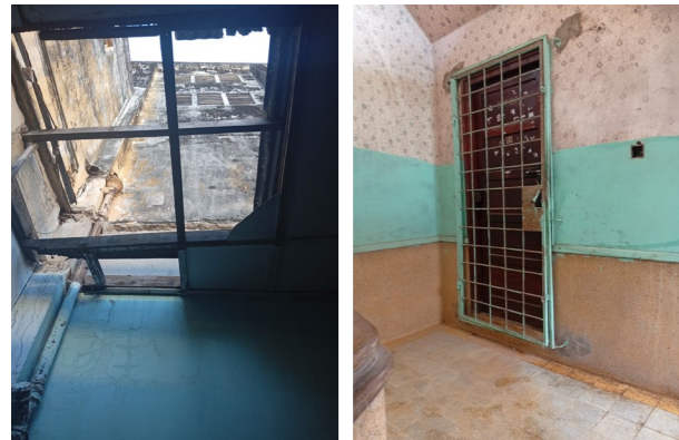
Fig67. The existing metal roof. View from groundfloor
