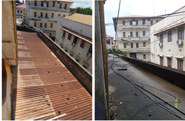
Fig65. The existing conjugated metal surface
