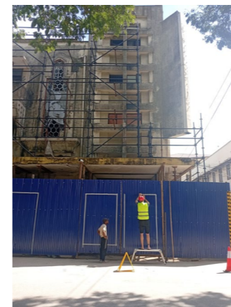
Fig50-52. Setting up the frames
