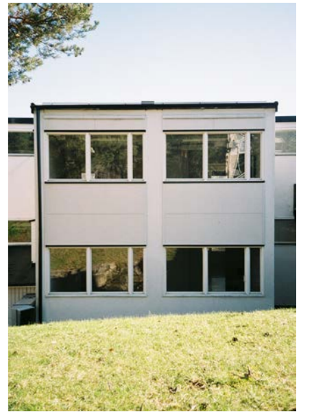
GROUP ROOM FACADE FIG. 31
