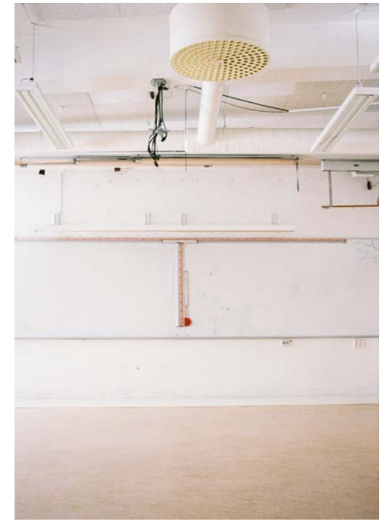
CLASSROOM II FIG. 53
