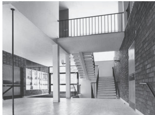
ENTRANCE, BUILDING A, 1956 FIG. 11
