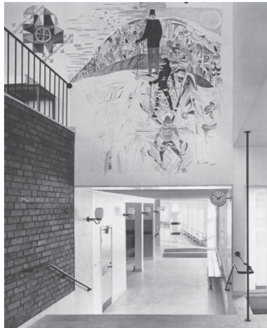
CORRIDOR, BUILDING A, 1956 FIG. 09
