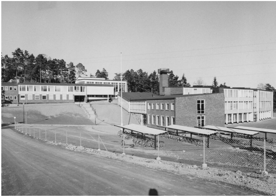
VIEW FROM THE HISTORICAL MAIN ROAD ACCESS
