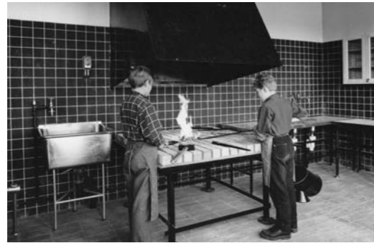
WORKSHOP, BUILDING C, 1956
