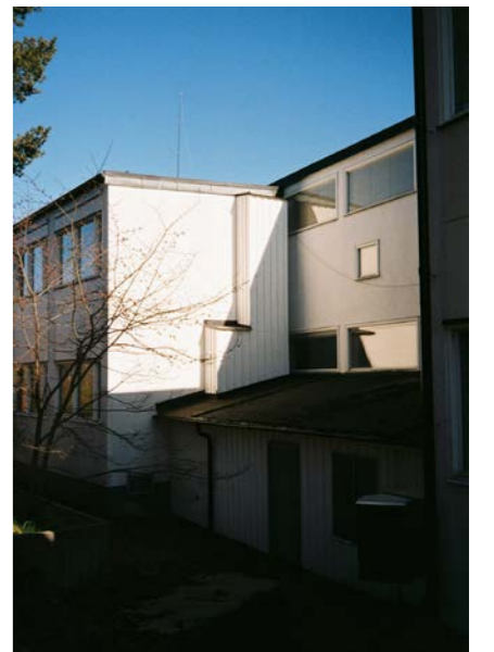
VENTILATION PAVILLION II FIG. 35
