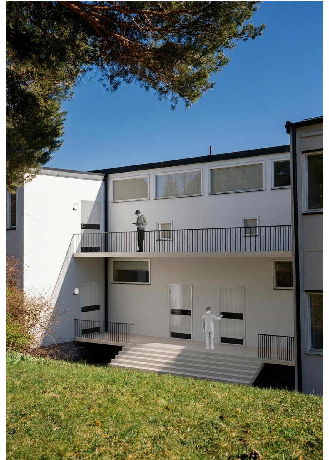
NORTH FACADE I
