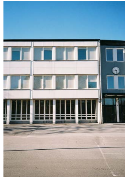
SOUTH FACADE FIG. 29
