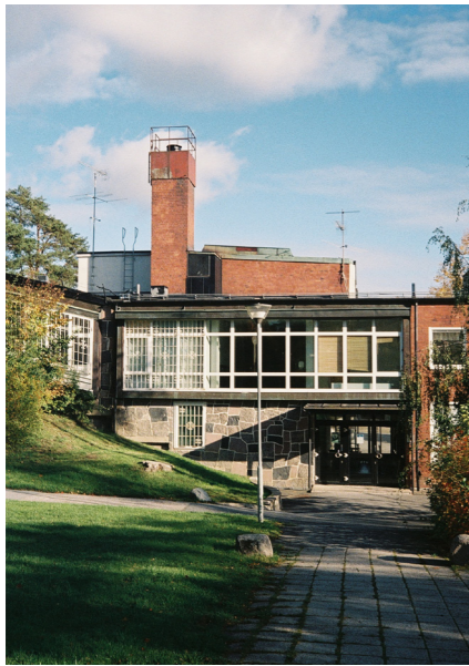
MAIN ENTRANCE I FIG. 22
