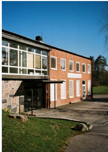
MAIN ENTRANCE II FIG. 26
