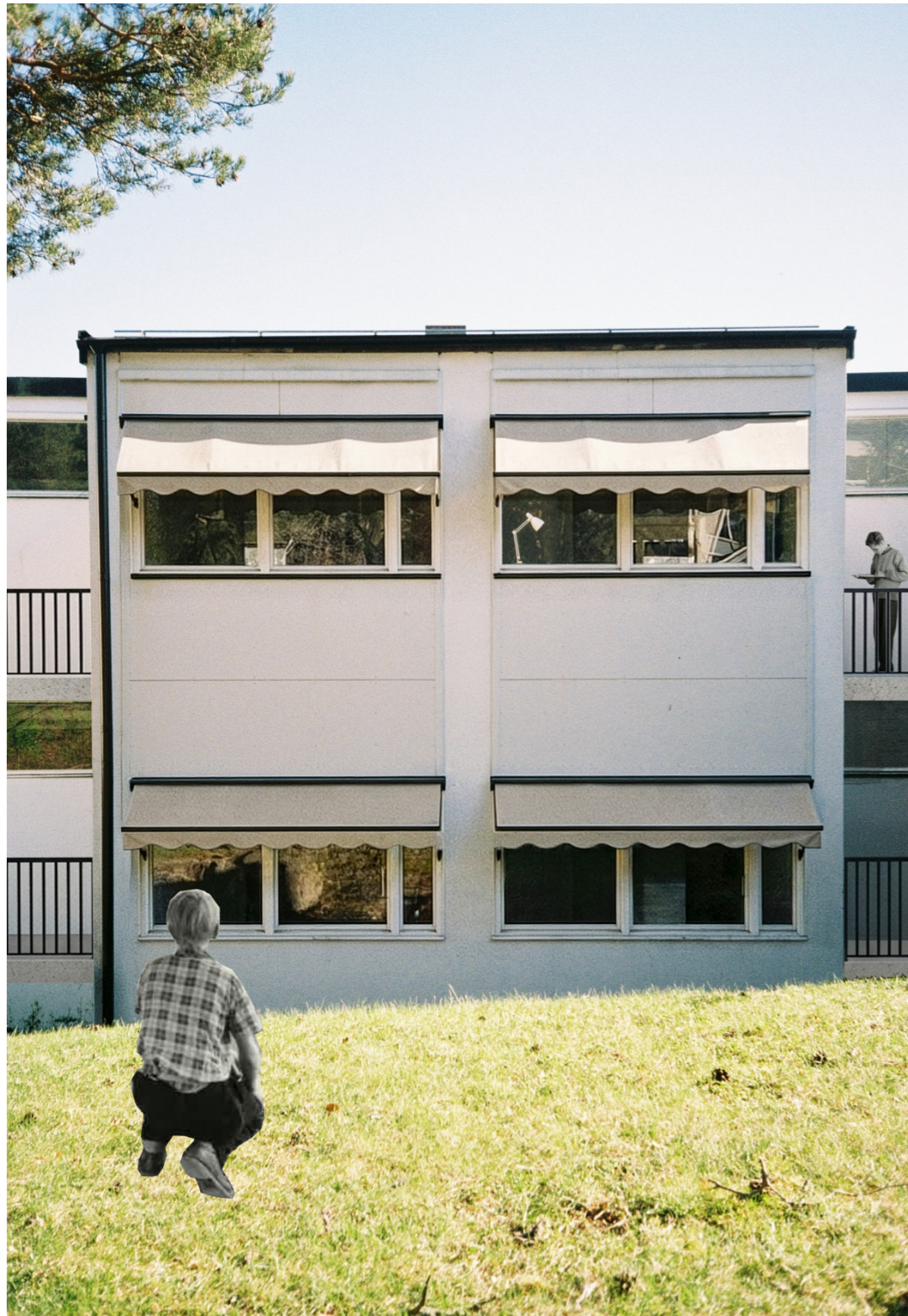
NORTH FACADE II
