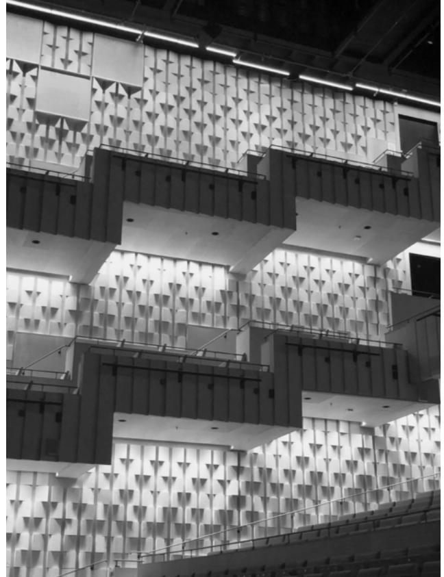
Figure 07. Sara Kulturhus: Wooden acoustic wall in concert hall. (Palmqvist, 2020). Published with permission.
