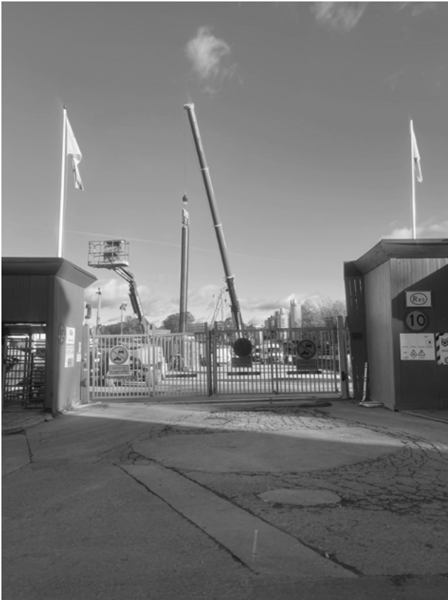
Figure 23. The construction site today. Author's own image.
