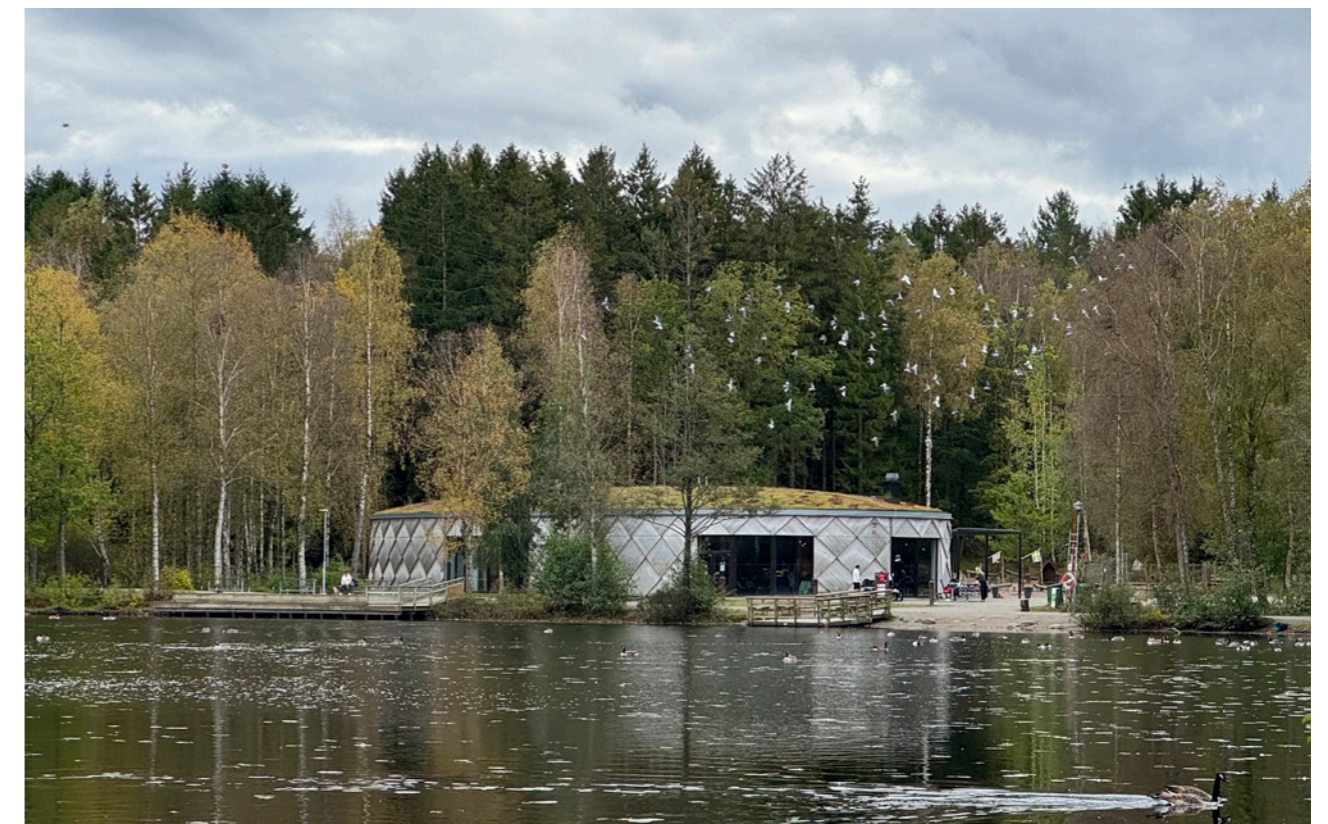
Figure 20. Motionscentralen Kotten by Tengbom.
