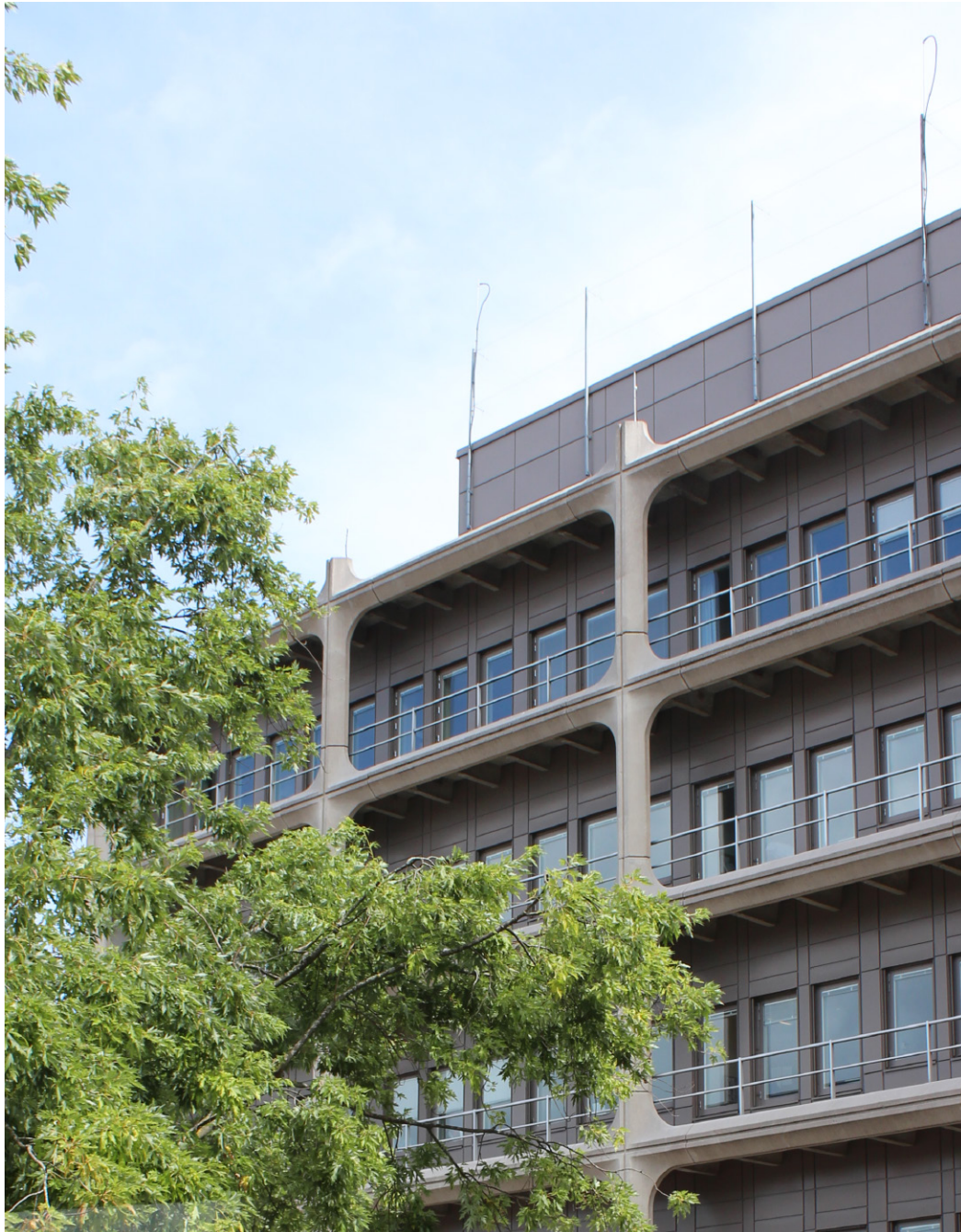
Figure 6. Facade toward northwest. One of few trees on site. (Author's photograph, 2025).
