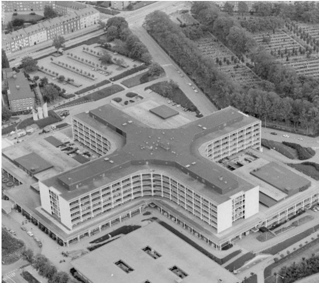
Figure 1. Aerial photo of Helsingborg Hospital. (Silverson, 1984).
