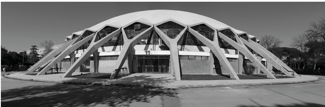
Figure 4 (Top). Ball stuck in the ceiling Palazzetto dello sport. (Absurdicus, 2014). CC-BY-SA 3.0 Figure 5 (Bottom). Outside of Palazzetto dello sport.
