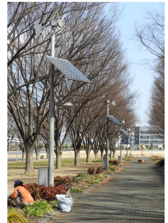
Figure A.6. Solar- and wind-powered street light, Tokyo Rinkai Disaster Prevention Park .
