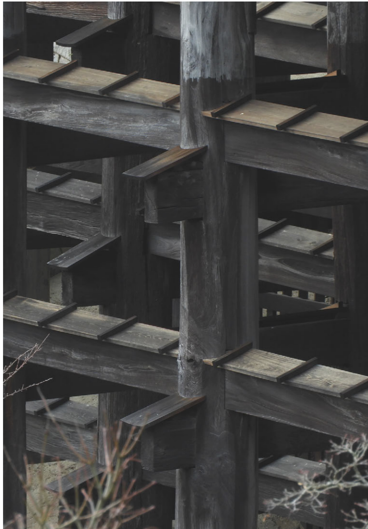
Figure 18. Kiyomizu-dera temple in Kyoto. The temple has endured for over a millennium thanks to the resilience of its wooden joinery, providing flexibility in earthquakes, and regular maintenance and reconstructions carried out by successive generations. In combination with its important cultural background, the temple has become a UNESCO world heritage site.
