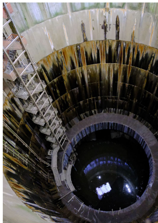
Figure A.3. One of the five water banks which is connected to the pressure-controlled tank,
