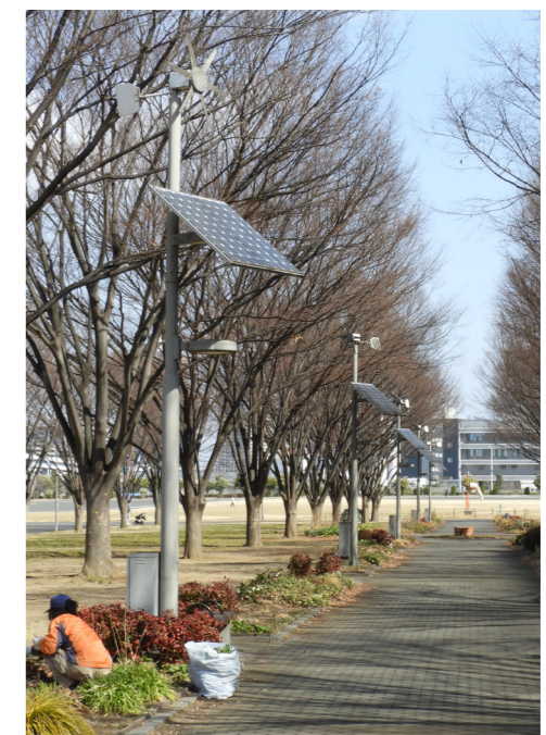
Figure 11. Solar- and wind-powered street light, Tokyo Rinkai Disaster Prevention Park .
