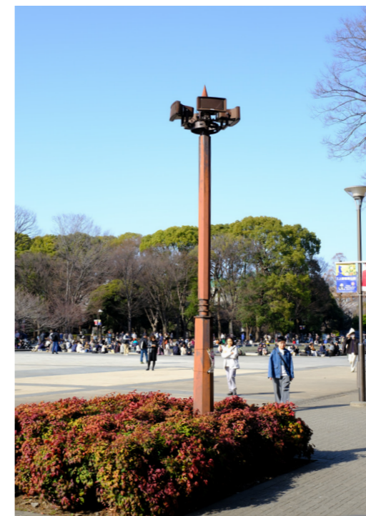
Figure A.7. Speakers used to broadcast information during times of crisis, Ueno park
