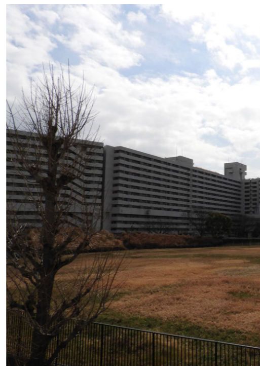
Figure A.4. Apartment complex acting as a fire wall to protect the park, Higashi-Shirahige.
