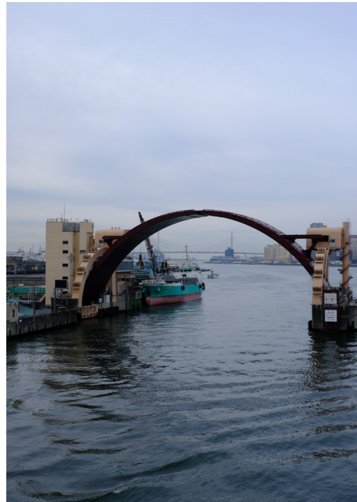
Figure A.1. One of five river sluice gates, Osaka.
