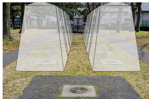
Figure A.19 Potholes for temporary toilets, Higashi-Shirahige.
