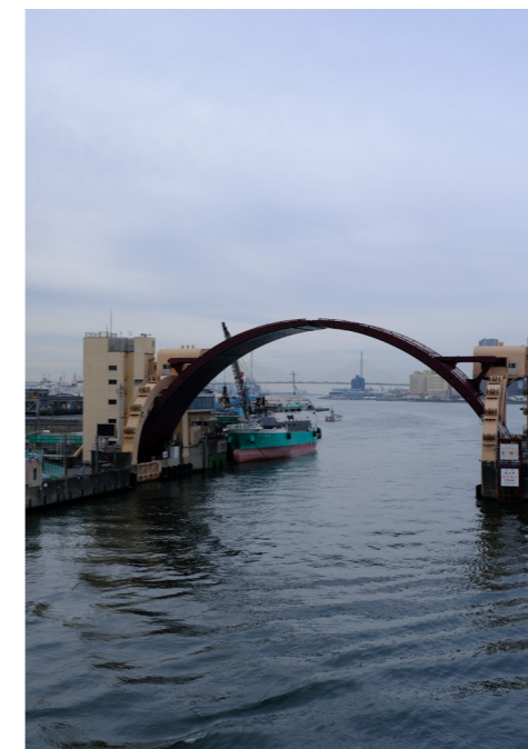
Figure 7. One of five river sluice gates, Osaka.
