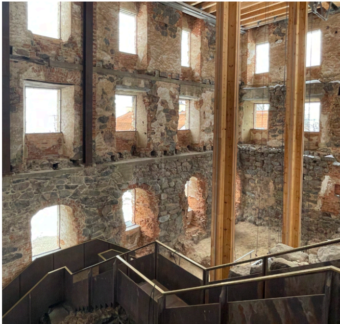
Fig. 11 Interior view of the castle, ceiling aligned with the former attic floor encasing the living volume.
