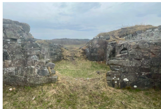
Fig. 45 Wall opening. Photo by author.
