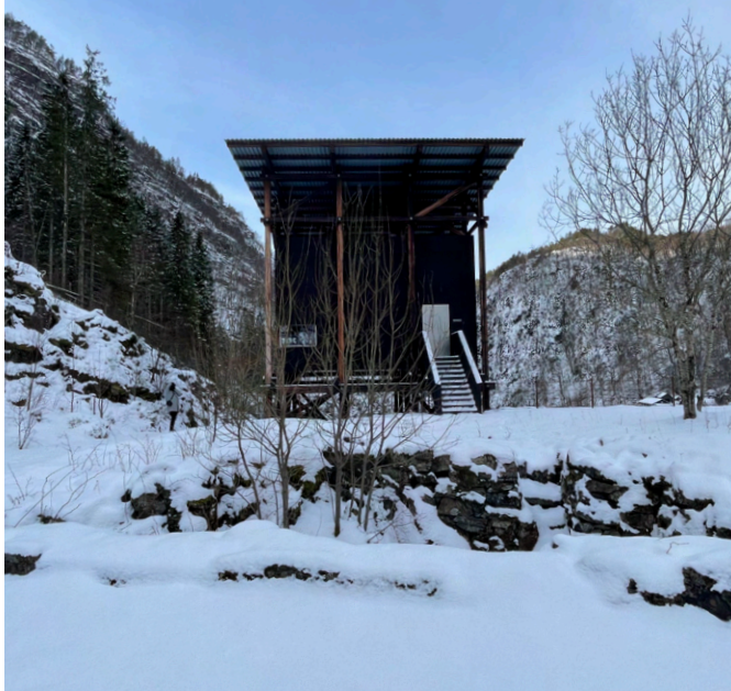
Fig.3 Cafe buildings inversion aligning with remains of the cellar of the mine adminstration building in foreground.
