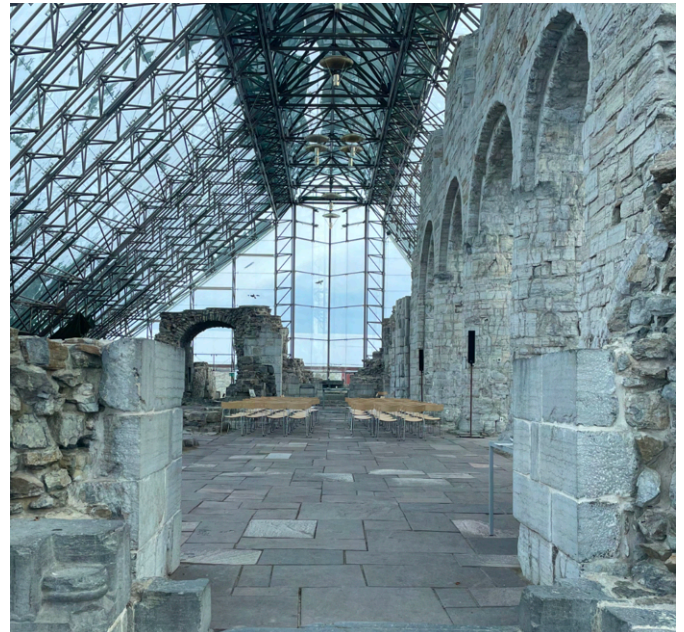
Fig. 10 Interior view. The Enveloping structure traces the perimeter of the site, not touching the remains.
