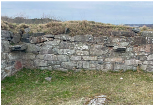
Fig. 42 Stone corbels. Photo by author.
