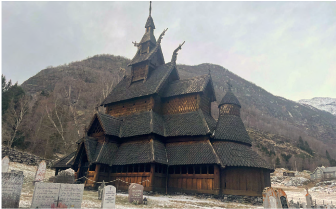
Fig. 23 Exterior view of Borgund stave church. The wooden structure through careful and continual repairs results in slow longterm decay.
