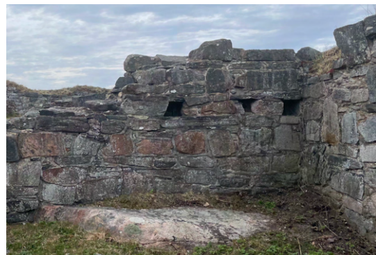
Fig. 43 Joist holes in wall. Photo by author.
