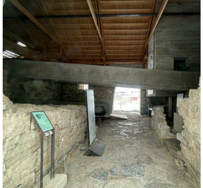
Fig. 8 Interior view of passage to courtyard with concrete walkway cutting across mid air.
