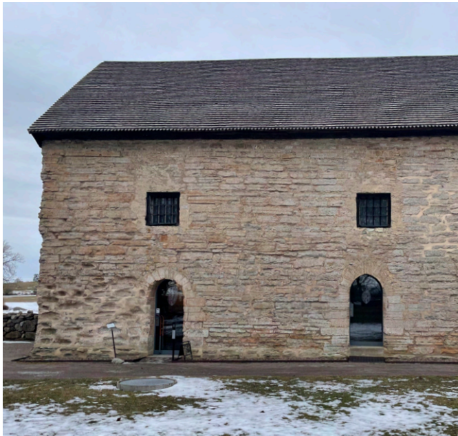
Fig. 15 Exterior view, carefully fitted glass doors do not disturb the exterior expression of the granary.
