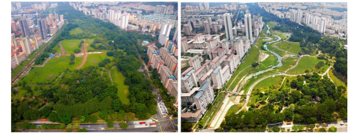
Fig 9: Before and after aerial view of Kallang River, Bishan Park, Singapore. (Pagodashophouse, 2011). CC BY-SA 3.0
