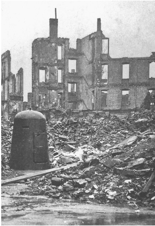
Fig. 7. A one-man bunker in Darmstadt withstood the fire. Stadtarchiv Darmstadt, with permission.
