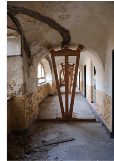
Figure 55: Structural supports in the barracks corridors
