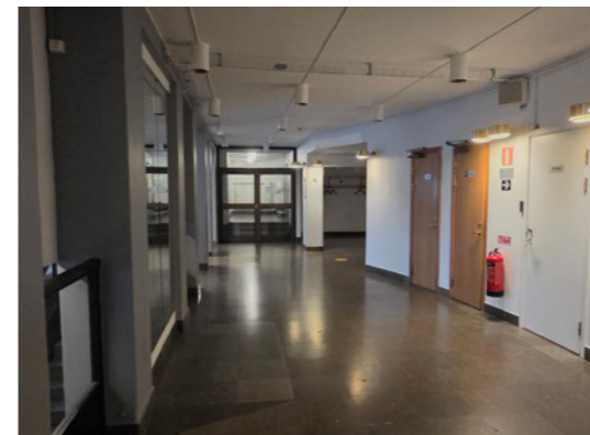
Figure 73. The foyer in its existing state.
