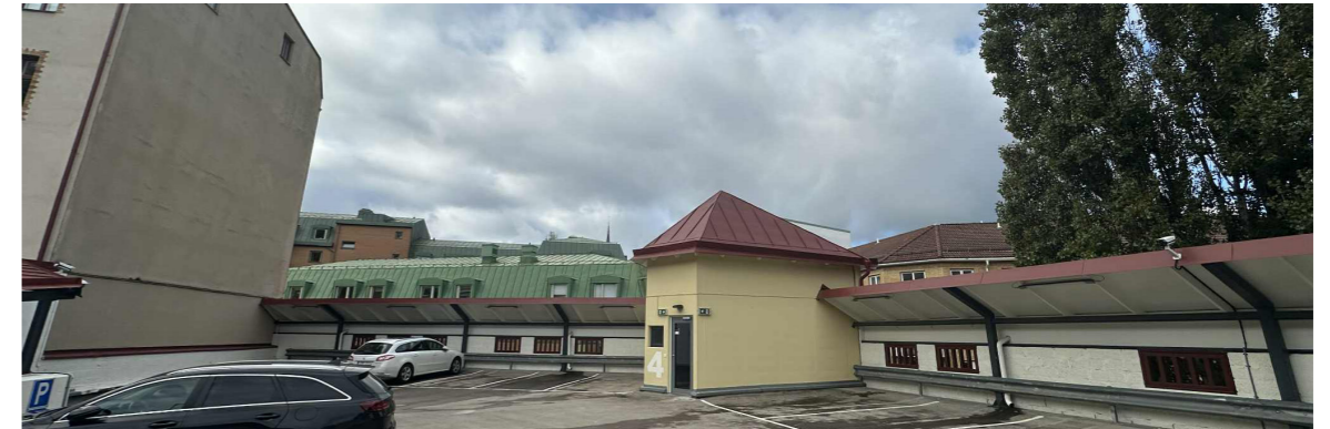
Figure 55: 4A - Looking West
