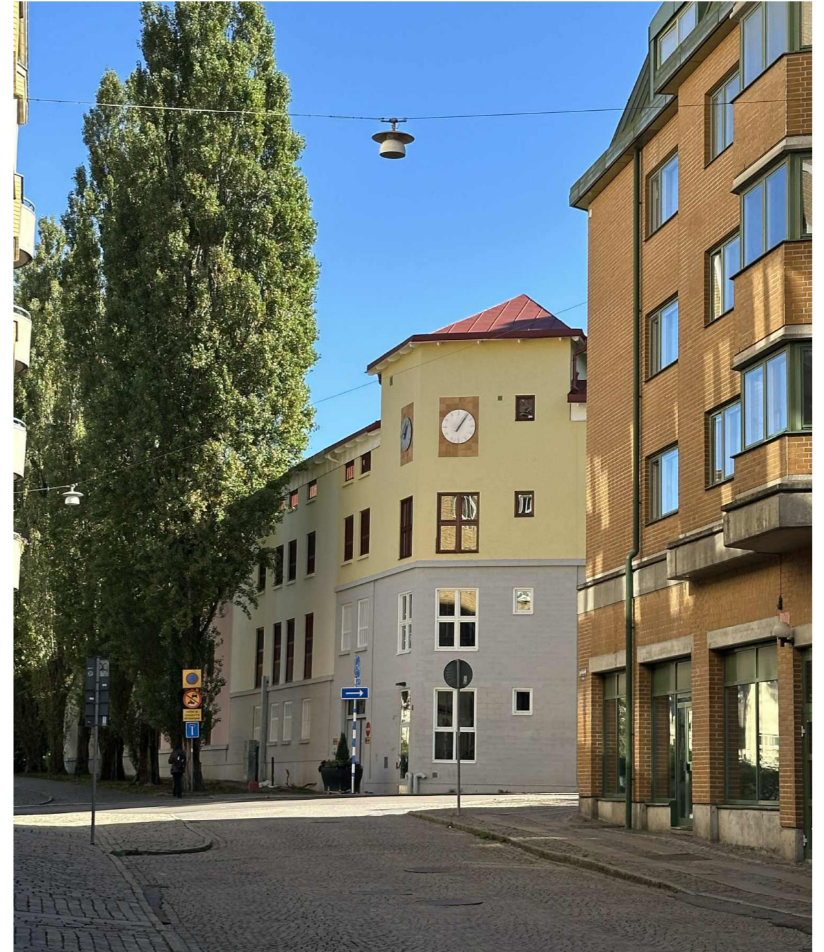
Figure 30: Authors Image - Street View 2025: Bergsgatan 3
