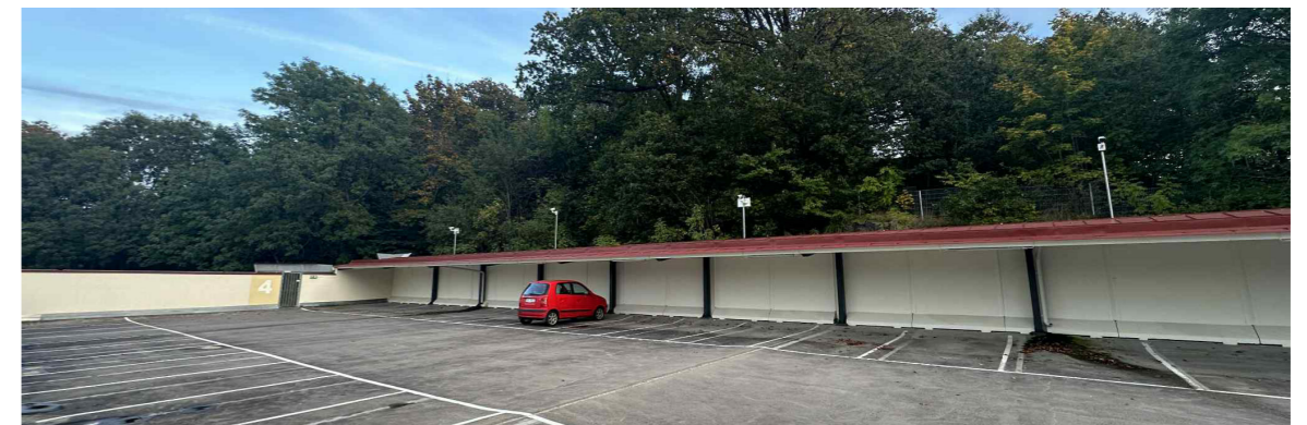
Figure 56: 4B - Looking South East
