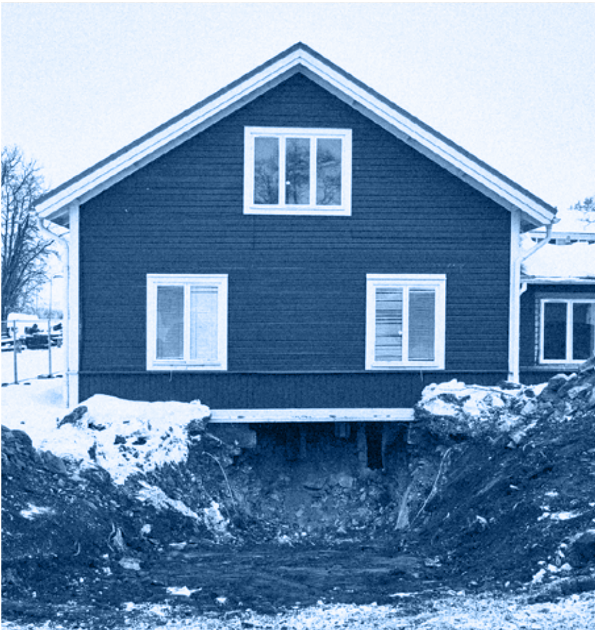
Fig. 49 Preparation for Movement of Arbetarbostaden B, 2017
