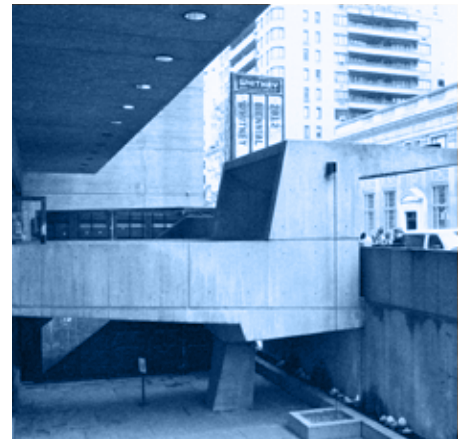
Fig. 62 Whitney Museum, Bridge Trench
