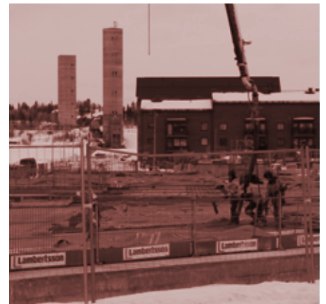
Fig. 03 Standard Concrete Construction
