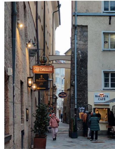
Material of building facades are natural stones.
