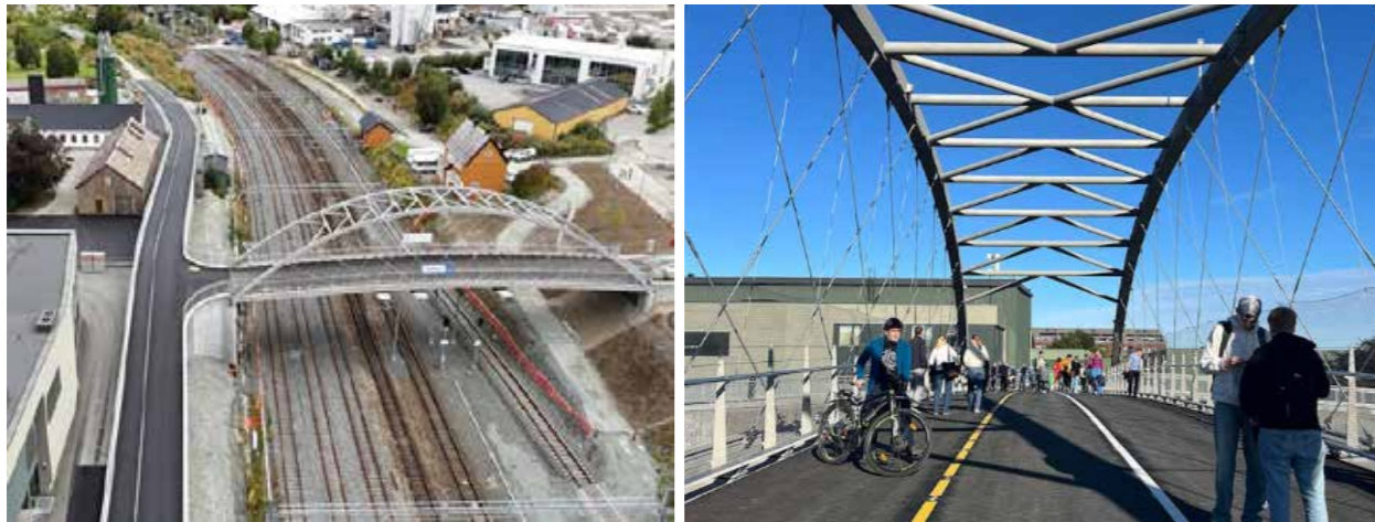
Figure A: Hangarbrua going across the railroad tracks at Leangen station in Trondheim, Norway. (Photo credits: Vegard Thorvaldsen/Statens vegvesen)
