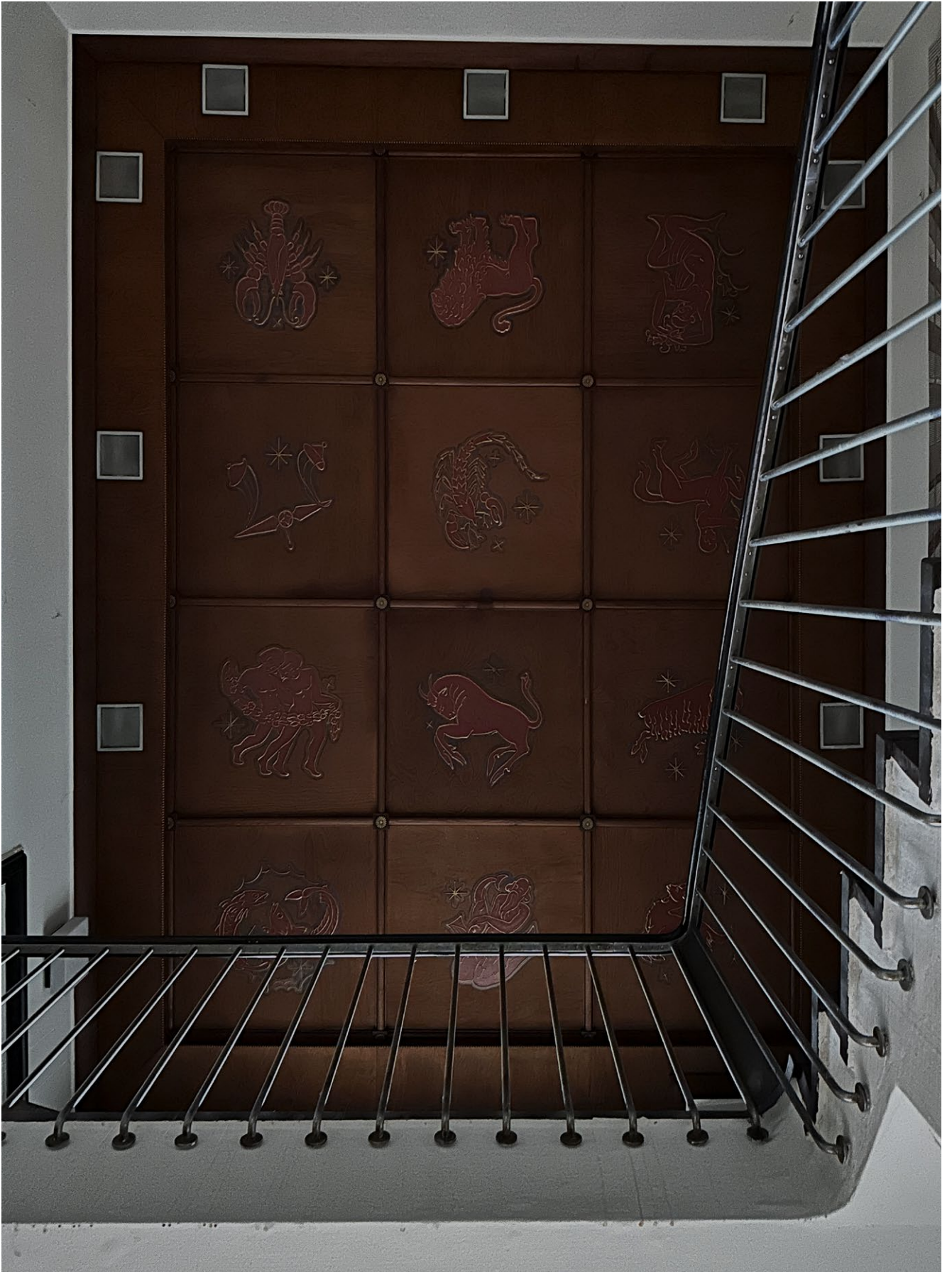
[Figure 39] - Original Ceiling Remnant, Main Entrance from Nobelvägen (Authors, 2026)
