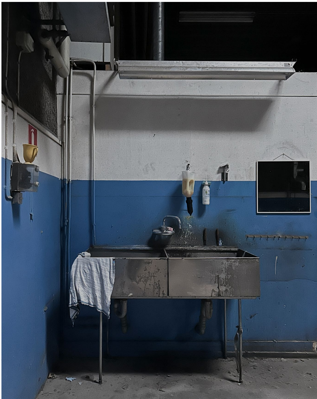
[Figure 24] - Usage Remnants, Industrial Hall (Authors, 2026)
