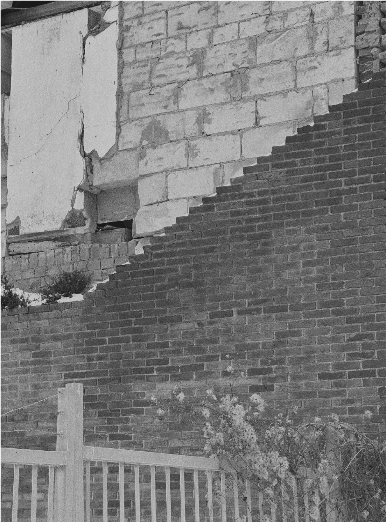
[Figure 2] - Ongoing Demolition, Östra Farmvägen, Malmö (Photo: Authors, 2026)
