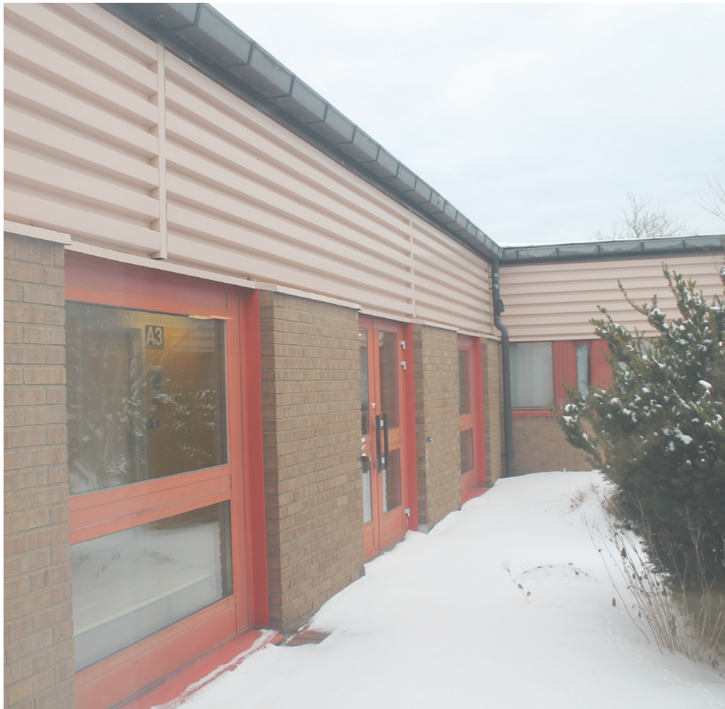
View from the inside courtyard of building 21
