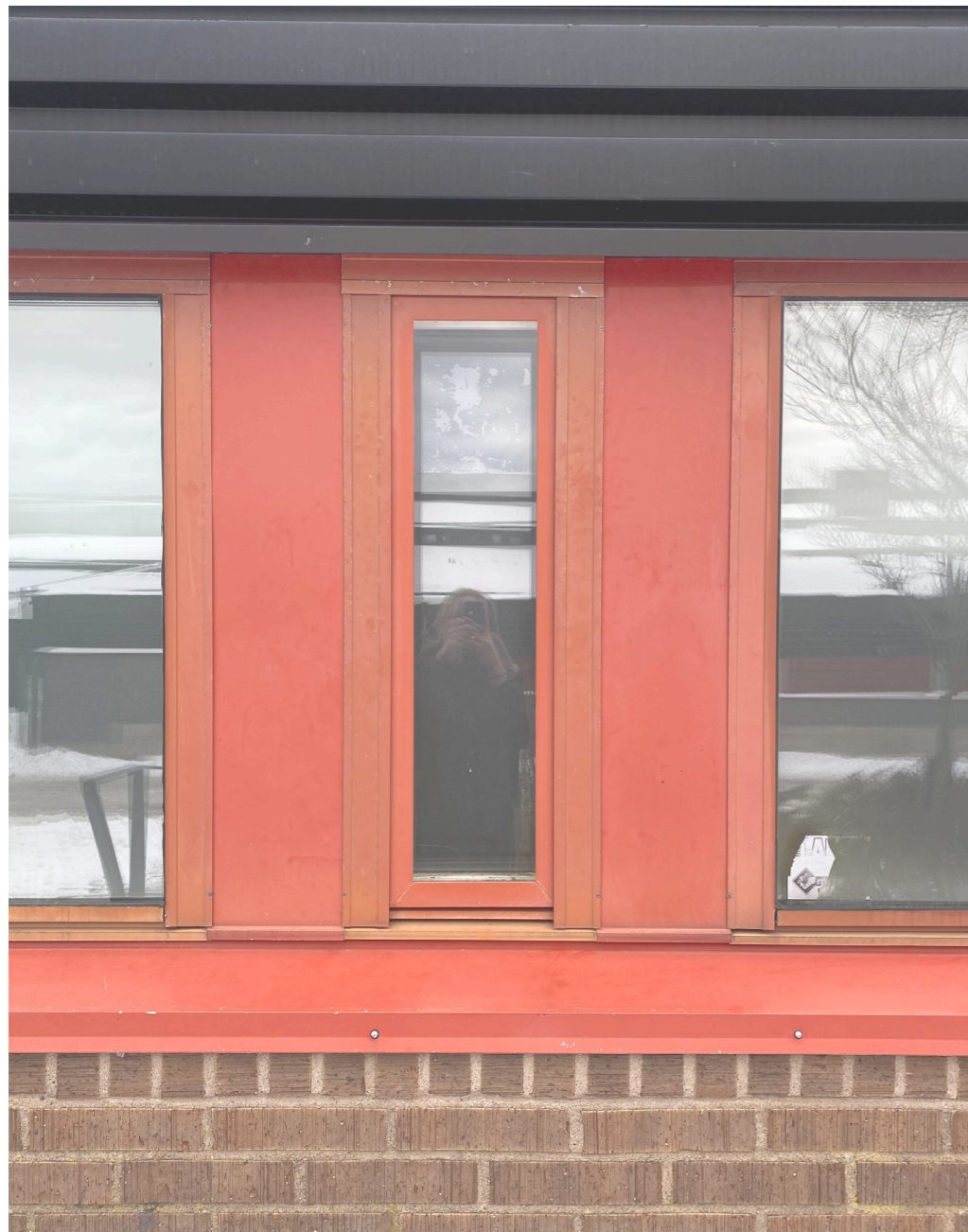
Exterior view of building 21
