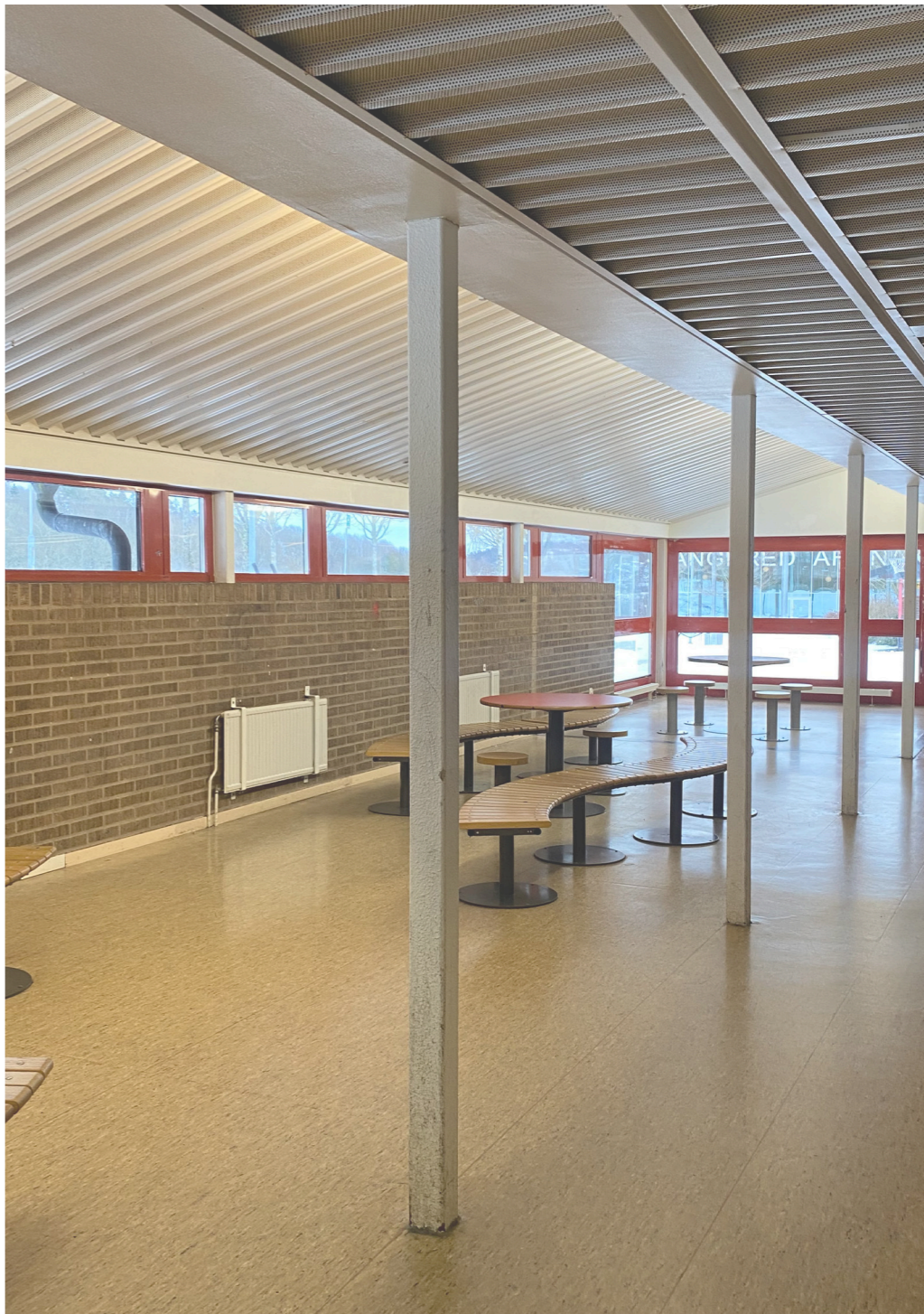
Interior View of Building 21
