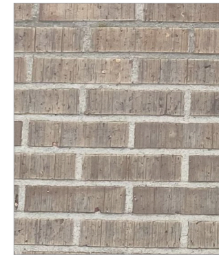
Material: Brick Category: 02. Envelope Reuse Potential: Challenging
