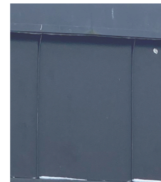
Material: Corrugated Steel Category: 02. Envelope Reuse Potential: Easy
