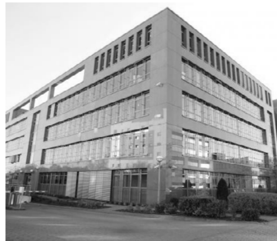
Figure 15: Existing façade of Da Vinci Source: Author
