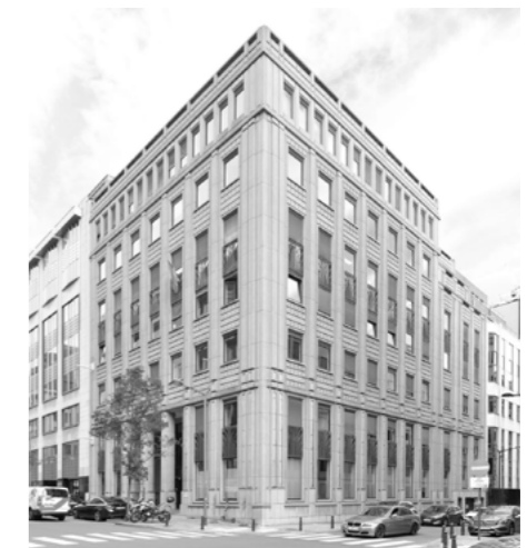
Figure 12: Existing facade of Montoyer 40 Source: Author
